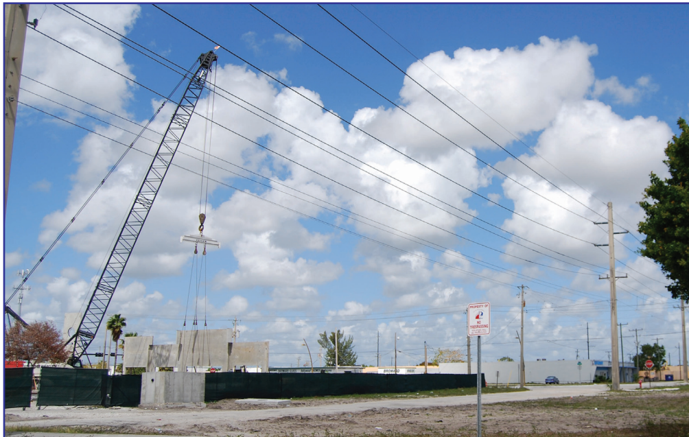
Shoppes on Avenue of the Arts Construction
