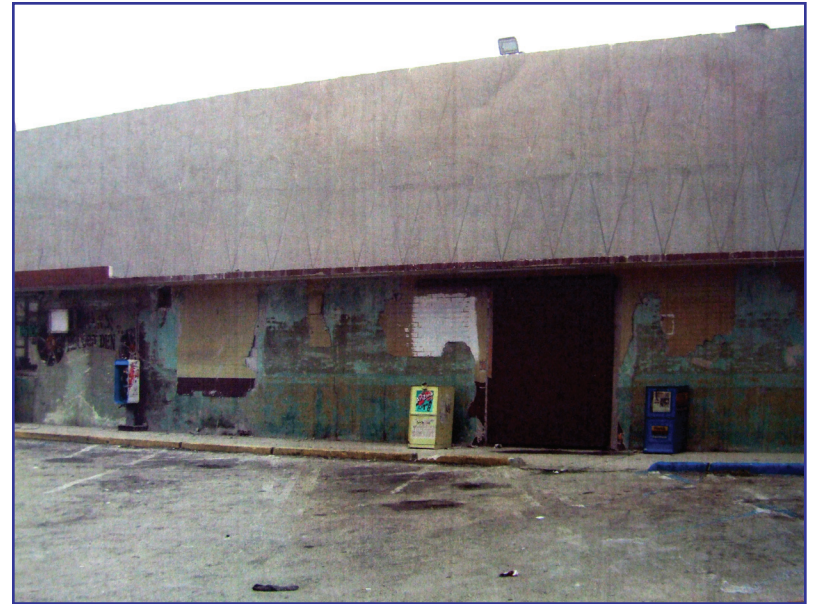
Bass Bros. Supermarket Façade - Before
