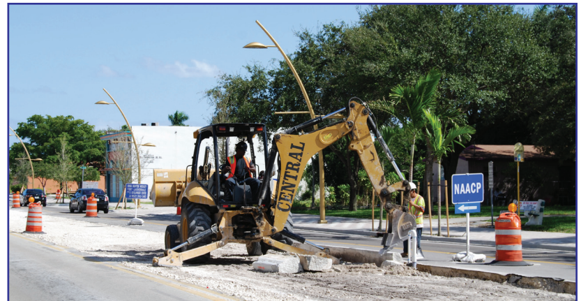
Sistrunk Boulevard Infrastructure Project Construction
