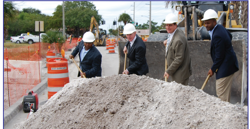
Sistrunk Boulevard Infrastructure Project Groundbreaking - Jan. 2011
