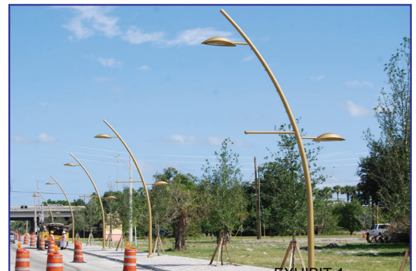
Sistrunk Boulevard Streetscape Lighting
