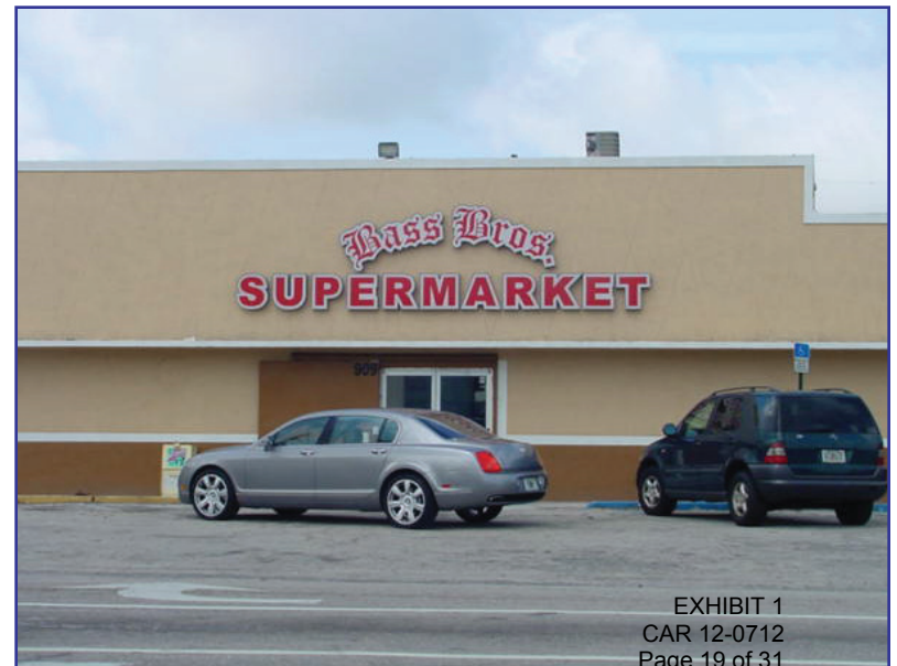
Bass Bros. Supermarket Façade - After
