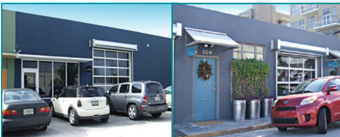
CRA Façade Program Improvements in FAT Village Arts District - 504 and 525 NW 1 Avenue
