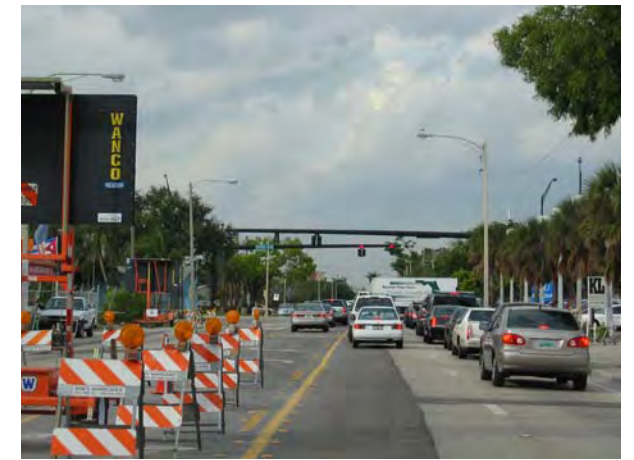
Construction along Andrews Boulevard
