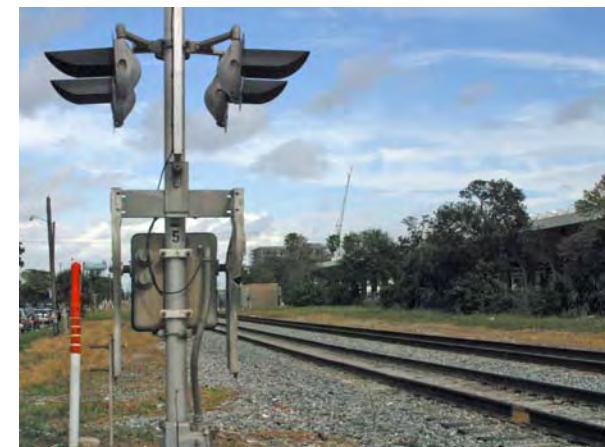
Rail line on the east side of the CRA project area
