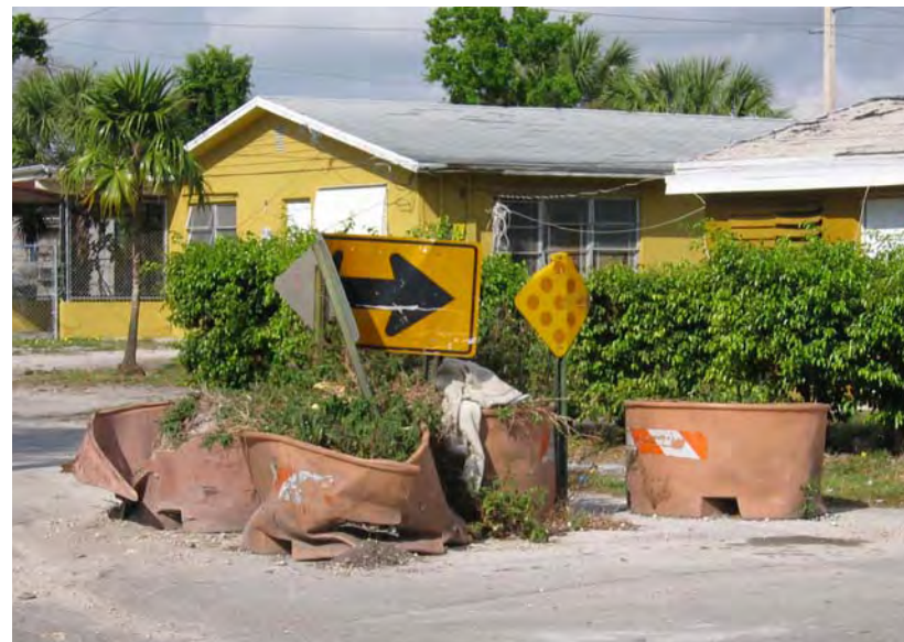
Existing conditions with traffic barriers
