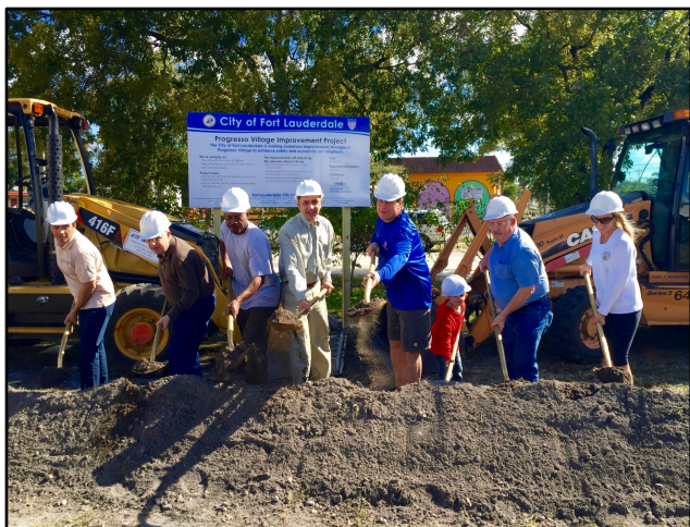
Commissioner Trantalis and Mayor Jack Seiler help residents of the Progresso Village neighborhood break ground on an improvement project that includes new sidewalks, swales, storm drains and lighting.
