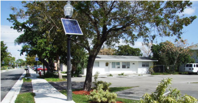
Phase II - NW Neighborhood Improvement Capital Project
