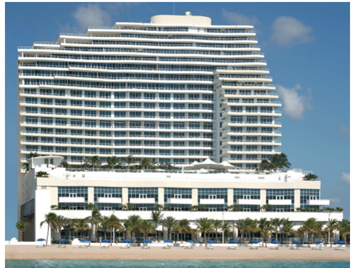
Renovation of the Ritz Carlton Hotel
