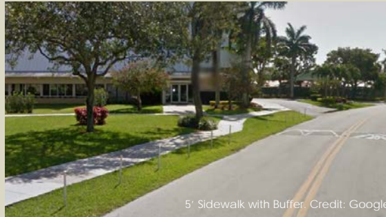
5' Sidewalk with Buffer. Credit: Google
