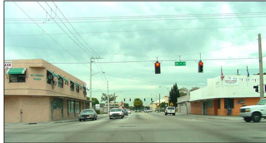
Figure 3.4, Sistrunk/NW 6 th Street Prior to Corridor Improvements
