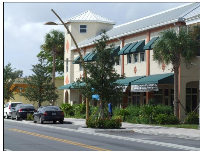
Figure 3.5, Sistrunk Boulevard/NW 6 th Street after Corridor Improvements
