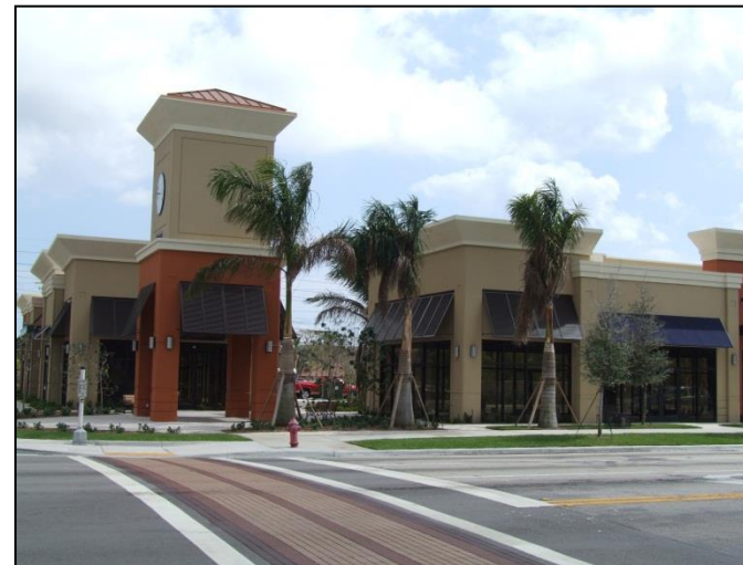
Figure 3.6, Sistrunk Boulevard/NW 6 th Street after Corridor Improvements
