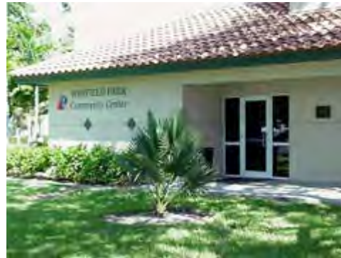
Figure 3.4 – Warfield Park Community Center
