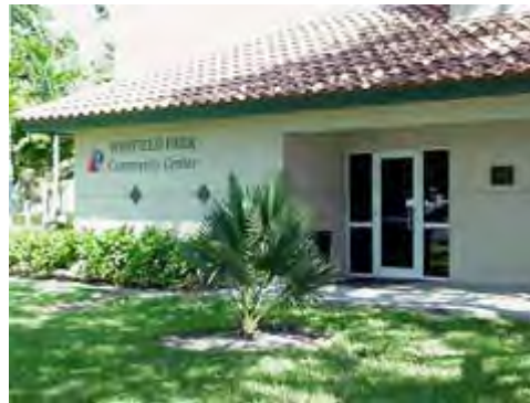
Figure 3.4 – Warfield Park Community Center
