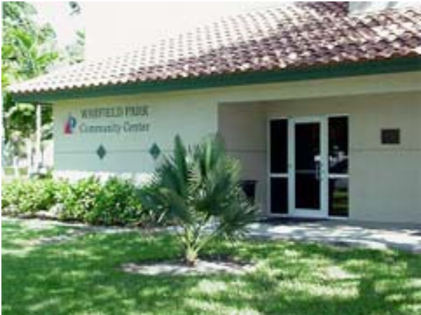
Figure 3.4 – Warfield Park Community Center
