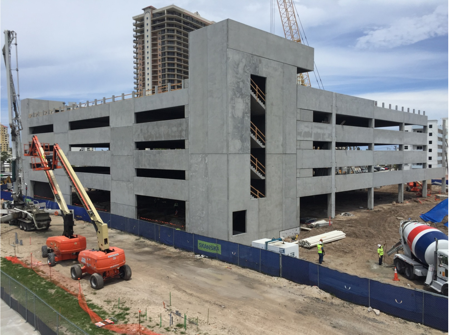
GARAGE PROGRESS PHOTO TAKEN ON 4-24-2018
