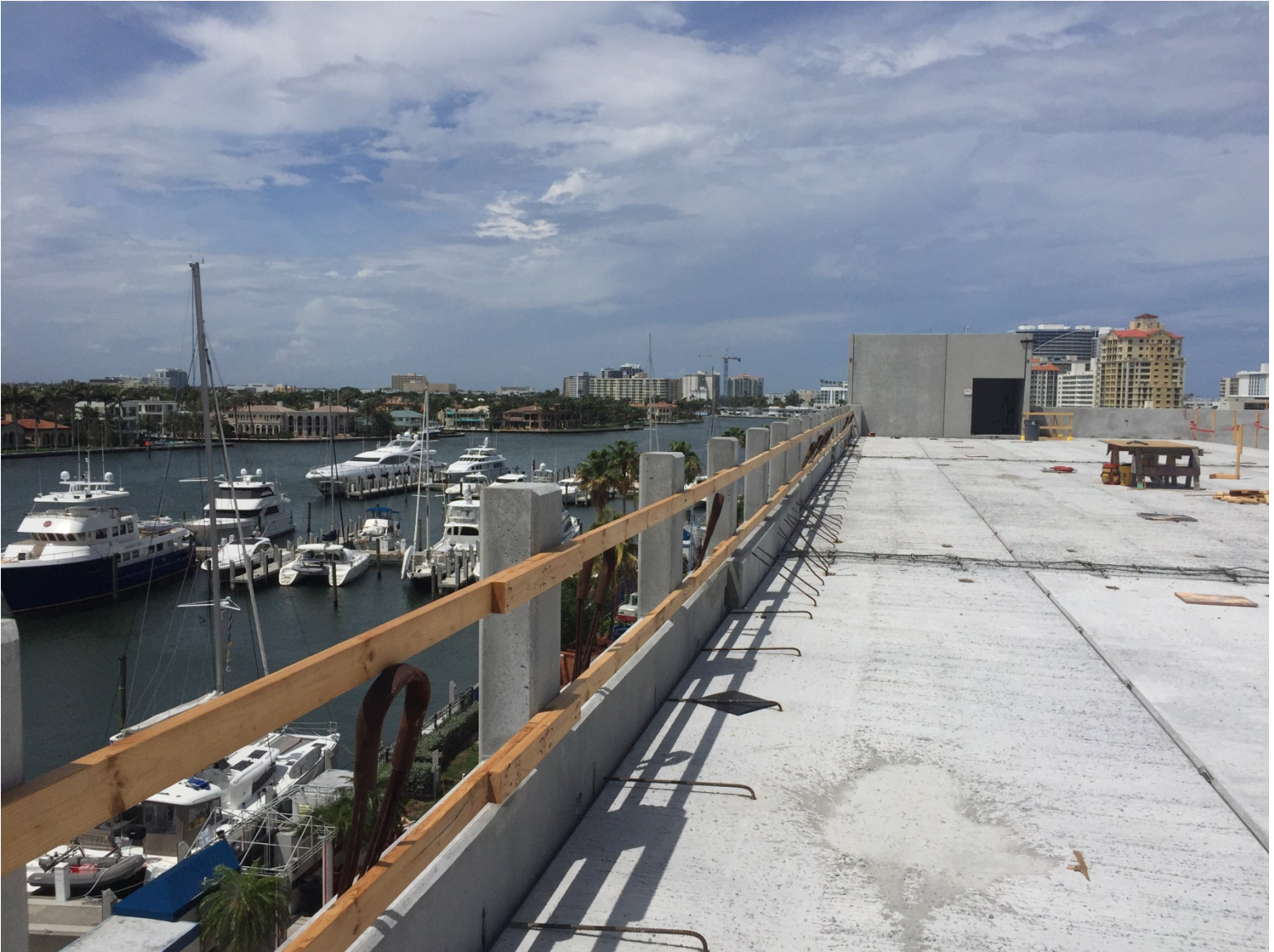
GARAGE PROGRESS PHOTO TAKEN ON 4-24-2018
