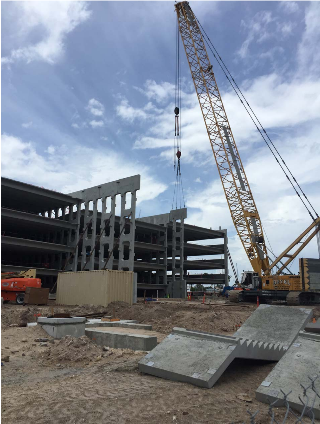
GARAGE PROGRESS PHOTO TAKEN ON 4-24-2018
