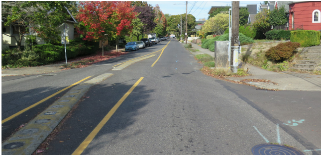
Off-set intersection bicyclist left turn median diverter
