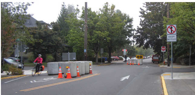
Partial closure - interim, stop-control
