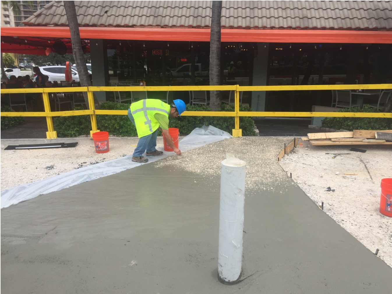
LAS OLAS BLVD PROGRESS PHOTO TAKEN ON 6-13-2018
