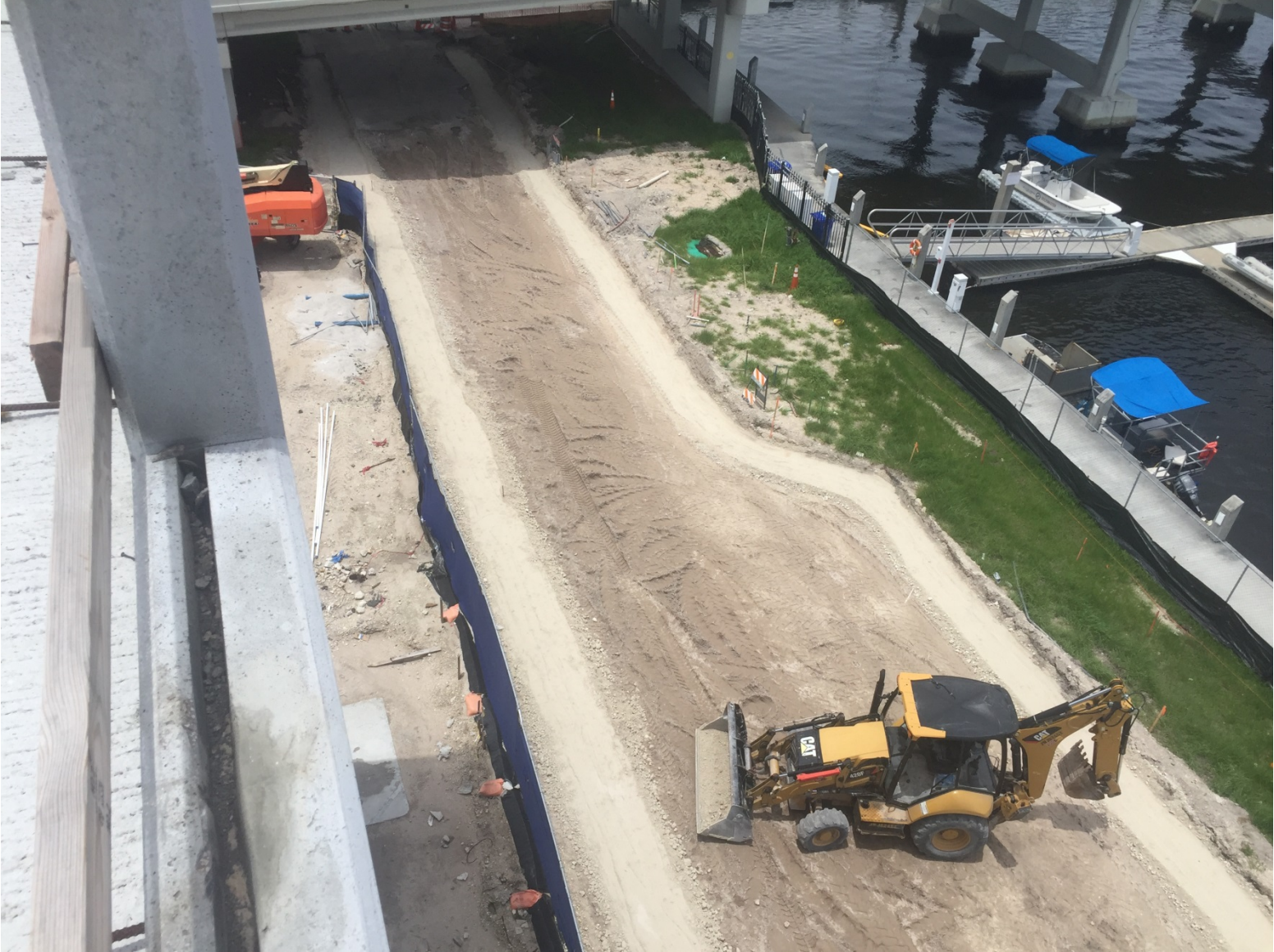
LAS OLAS CIRCLE PROGRESS PHOTO TAKEN ON 6-13-2018
