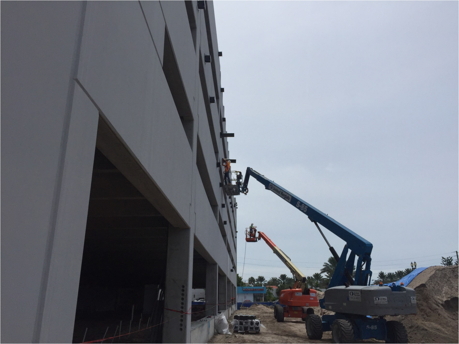
GARAGE PROGRESS PHOTO TAKEN ON 6-13-2018
