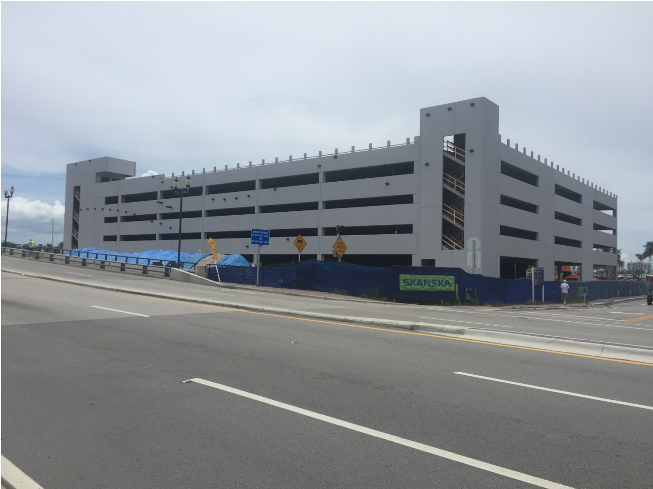
GARAGE PROGRESS PHOTO TAKEN ON 6-13-2018
