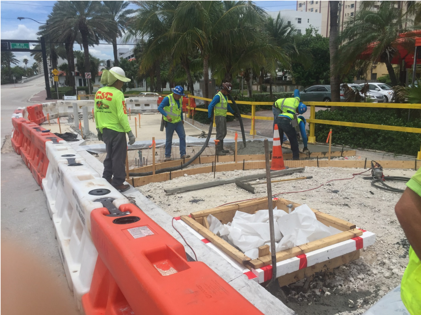
LAS OLAS BLVD PROGRESS PHOTO TAKEN ON 6-13-2018
