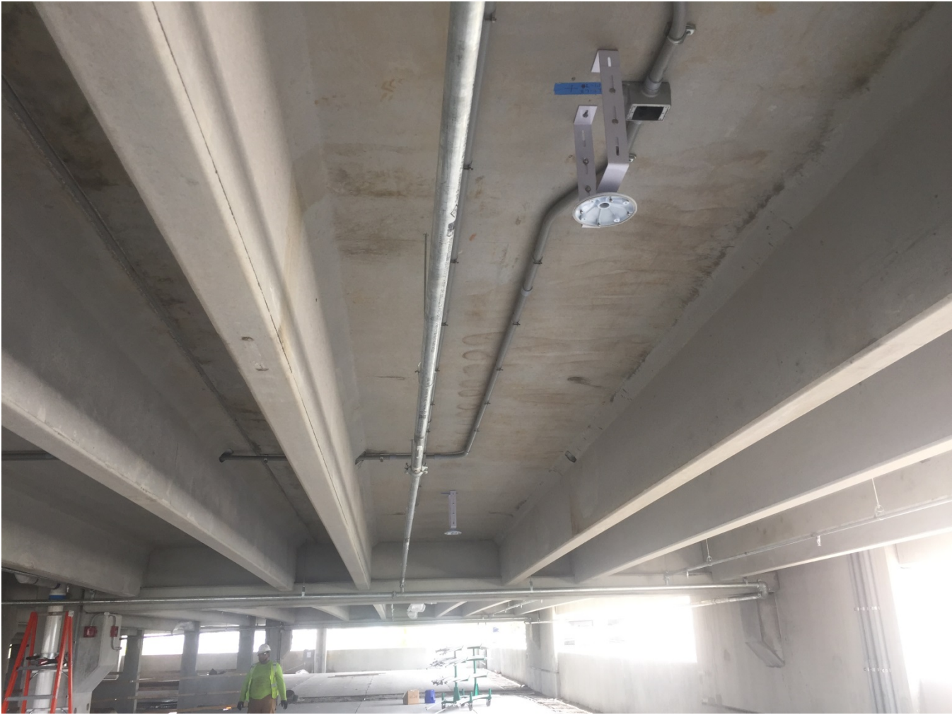
GARAGE PROGRESS PHOTO TAKEN ON 6-13-2018
