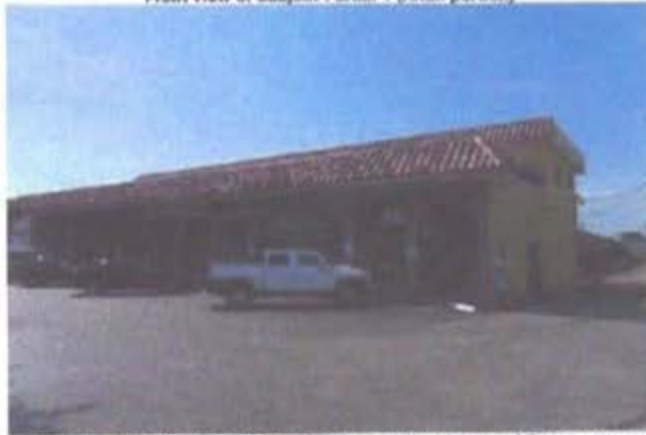
Front and west side view of Subject Parcel 1 (retail with second floor apartments)
