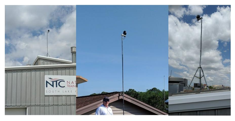
Our Lightning Sensors do not always have to be on the tallest building or object onsite, but need to have the best possible view of the sky in order to be able to accurately monitor the static electricity changing in the local atmosphere.
