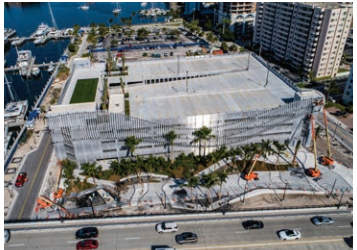
Las Olas Boulevard Parking Garage Construction
