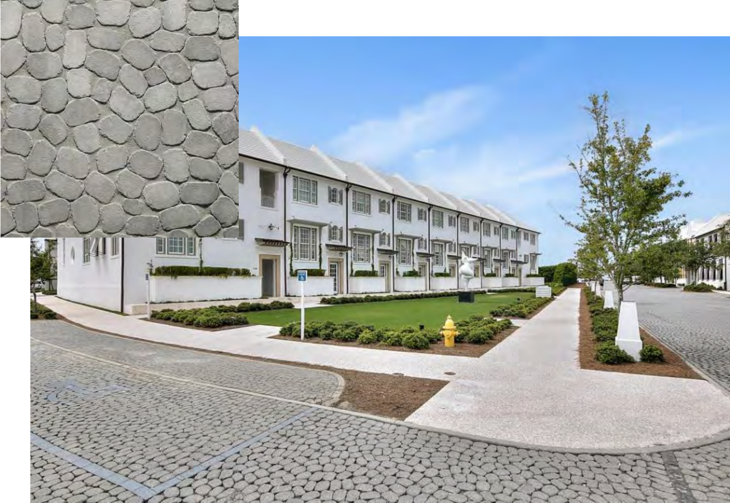
Roadway - Tumbled Concrete Pavers
