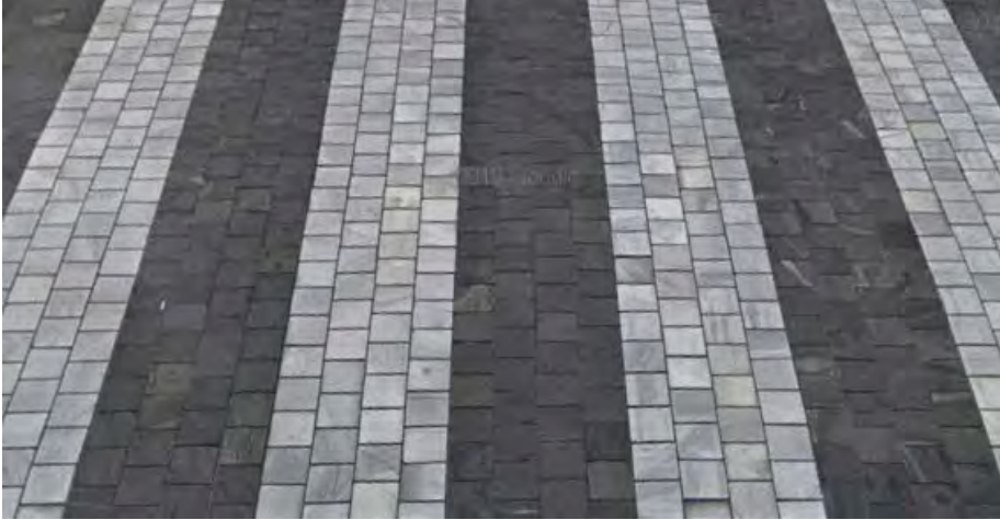
Rectangular Pavers for Crosswalk and Valley Gutter
