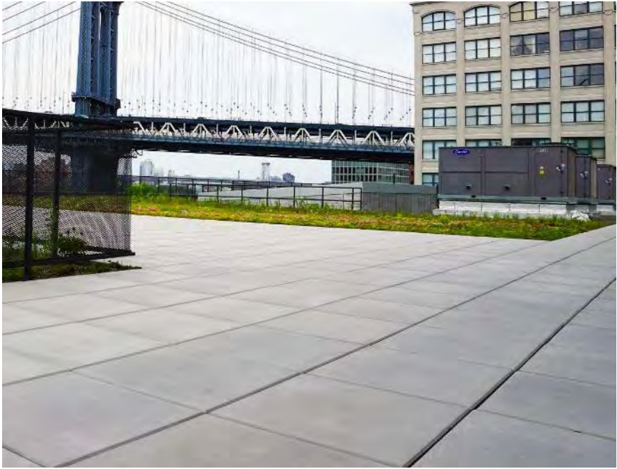
Sidewalk – Concrete Pavers
