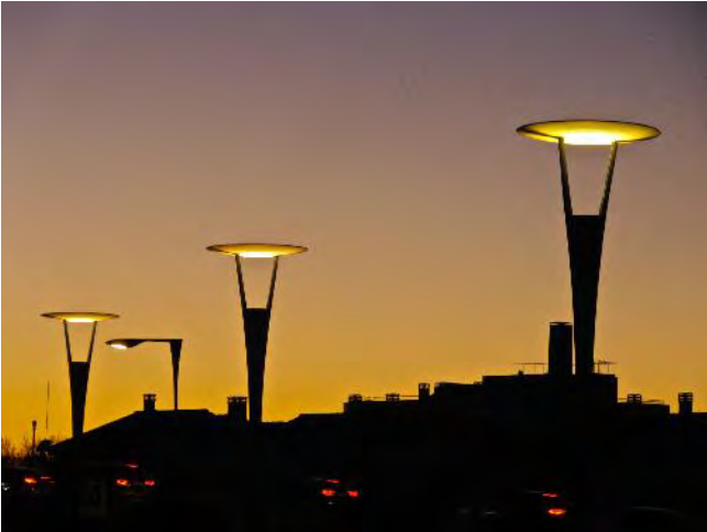
LED Street Lighting
