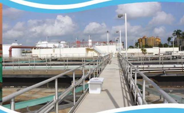
Secondary Clarifier Walkway
