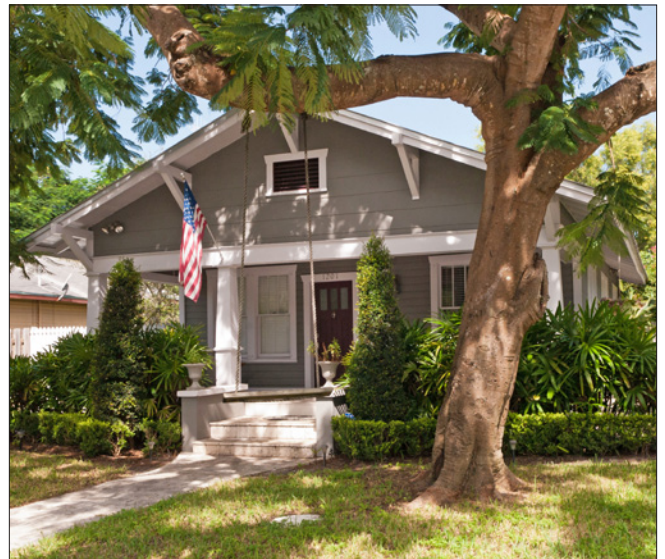
The Sailboat Bend Historic District includes a varied collection of residences of different architectural styles. This Craftsman Bungalow has a front gable roof with bracketed, deep overhanging eaves.
