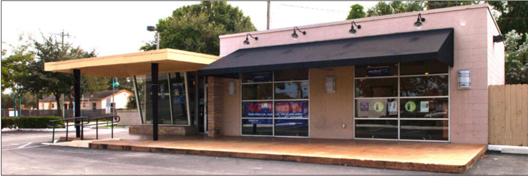
The HPB review process allows for flexibility for property owners and design professionals when approaching a project. This former service station has been adaptively reused as a retail store. The garage doors have been replaced with large fixed windows and an awning above.
