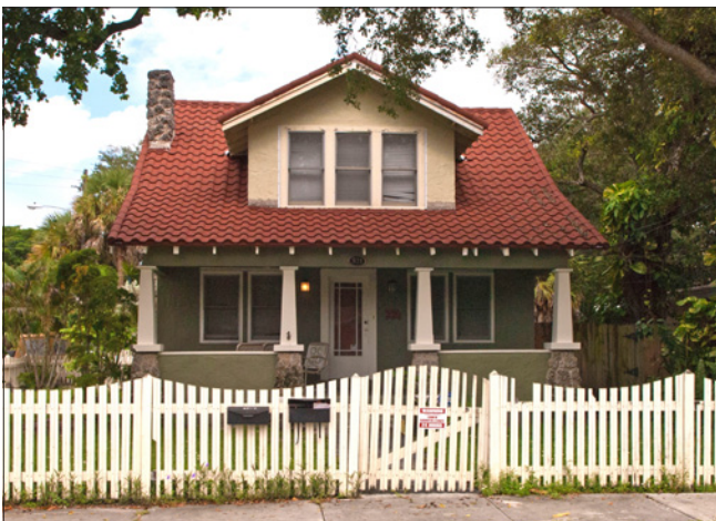
This masonry bungalow has a side gable tile roof with deep overhanging eaves. Also note the tapered porch piers, typical of the Arts and Crafts style.
