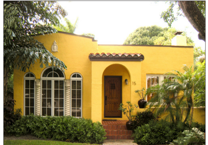
This modest Mediterranean Revival / Spanish Eclectic residence has a group of three arched window openings separated by turned mullions and a projecting entrance porch with a clay tile roof.
