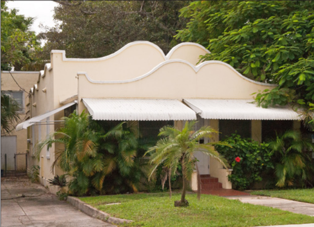
Mission Revival residences often have flat roofs with decorative parapets. In this case, the parapet detailing is located at both the main roof and projecting secondary roof.
