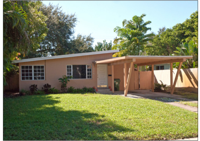
This Mid-Century Modern home has a shed roof, and asymmetrical facade and an attached, projecting, flat roof car port supported by narrow columns.
