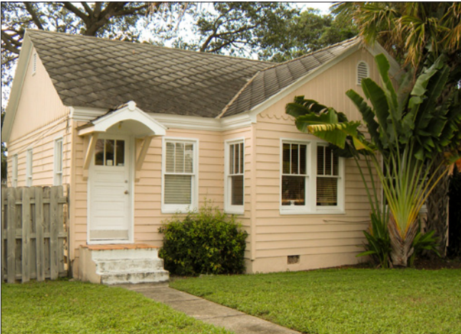
The exterior of this wood-framed "L"-shaped, residence is covered with wood clapboards, with the exception of the gable ends, which have vertical boards with scalloped ends.
