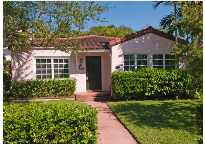
This "L"-shaped vernacular masonry house has a clay tile hipped roof with an intersecting gable roof. The form and materials are similar to the Mediterranean Revival style, although simplified.
