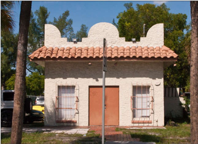
This small building has a stuccoed wall surface, a decorative Mission Revival parapet and is encircled by a hipped, clay tile, pent roof.
