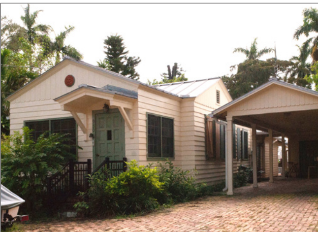
This shallow front-gable residence has a central cross gable and narrow eaves. The house is covered with wood clapboards, with vertical boards with scalloped ends at the gable ends.
