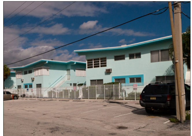
These Mid-Century Modern buildings have butterfly roofs that appear “folded” at their center. The projecting roof eaves provide shading for the wrapping corner windows.
