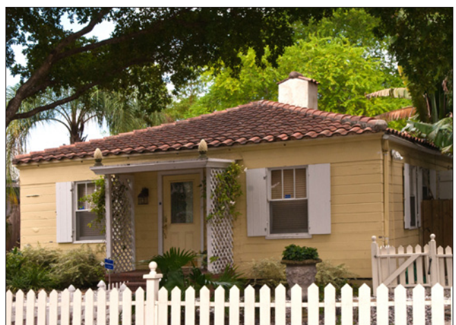
This wood framed residence has a hipped tile roof with shallow eaves and a central chimney. The symmetrical facade has an entrance door flanked by 3-over-1 double-hung windows.
