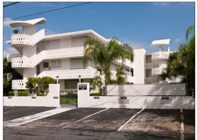
This Sub-Tropical Modern style apartment building includes covered wrapping balconies and exterior stairs that allowed circulation and provided shading for windows and doors.
