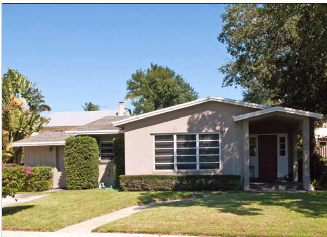
This masonry vernacular residence was constructed in the second half of the 20th century. It has a shallow pitched roof with overhanging eaves and grouped awning windows.
