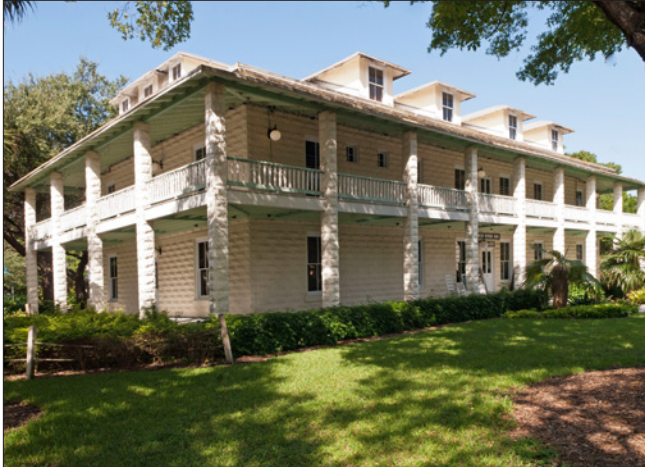
This 2-story, rusticated concrete block building has a wrapping second floor balcony covered by the main hipped roof and supported by rusticated concrete block piers.
