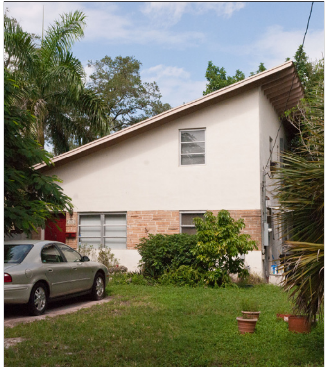
The dramatic shed roof of this Mid-Century Modern residence is an important character-defining feature that should be maintained if alterations are considered.
