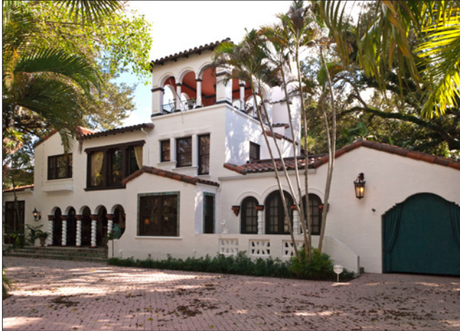
This Mediterranean Revival / Spanish Eclectic home has a central tower with an open belfry, an asymmetrical facade, and numerous grouped arch openings separated by decorative turned mullions.
