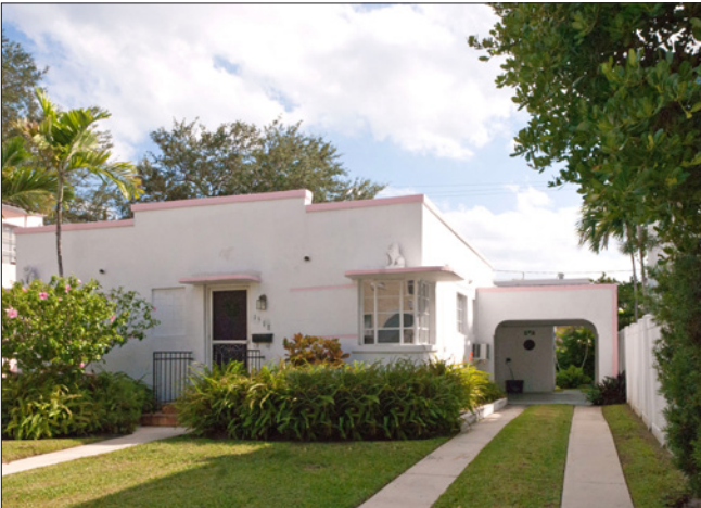
This Art Moderne residence has a central projecting parapet topped by a coping, corner wrapping windows with cantilevered sun screen, and a smooth stucco surface with horizontal grooves.
