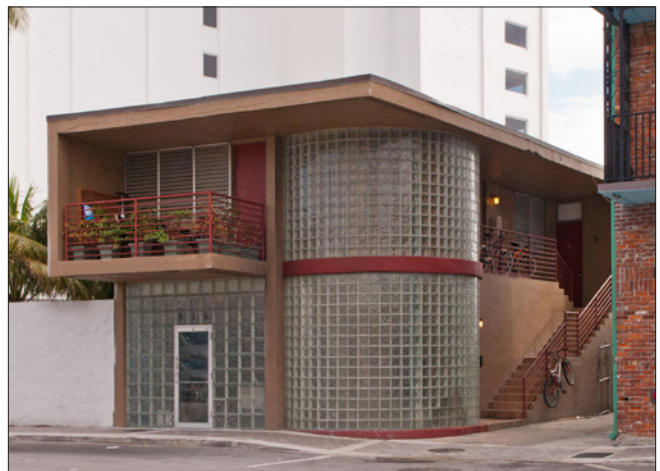
This Mid-Century Modern building has a semi-engaged, round, glass block corner and a projecting balcony under a unifying flat roof slab.
