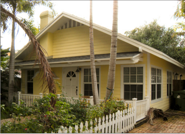
This wood framed vernacular house is 1-story in height, has a front gable roof with overhanging eaves, and has single and paired double-hung windows.
