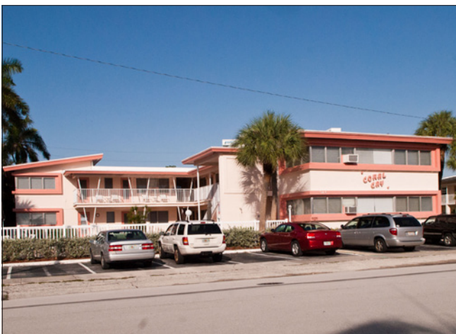
This Sub-Tropical Modern motel has projecting “boxes” framing ribbon window openings and covered balconies that allow for circulation and sun screening.
