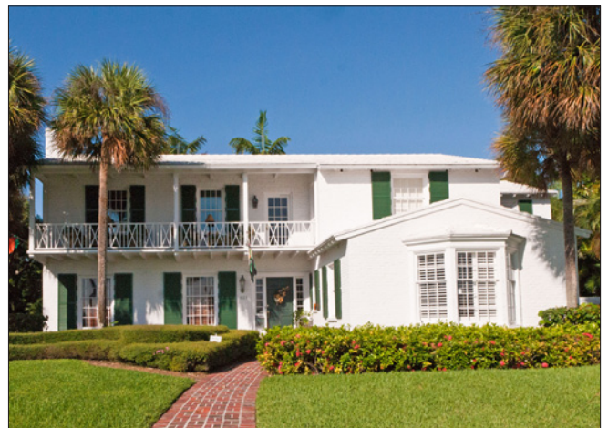
This Monterey style home has a shallow side gable roof that extends to cover a second floor suspended balcony. The 1-story section is a later addition.
