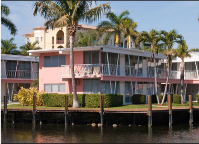
This is one of a group of Mid-Century Modern, 2-story, flat-roofed apartment buildings, each with a second floor balcony covered by the main roof, supported by narrow, angled “beanpoles”.
