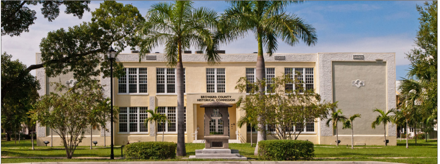
The West Side Grade School building, designed by architect John Morris Peterman in the Mediterranean Revival style, was constructed in 1922. It includes a flat roof with parapets and a stucco wall finish. The Harmon Monument, located at the center of the photograph in front of building, was originally a drinking fountain. The building now serves as the offices for the Broward County Historical Commission.
