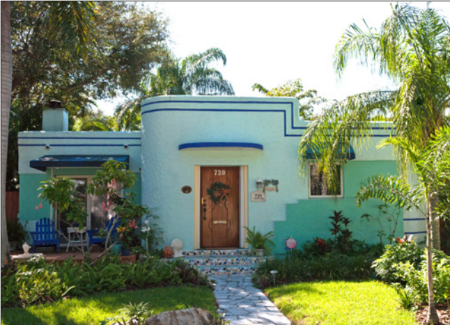
This residence has curved forms typical of the Art Deco period with decorative grooves and cantilevered sun screens over window and door openings typical of the Art Moderne period.
