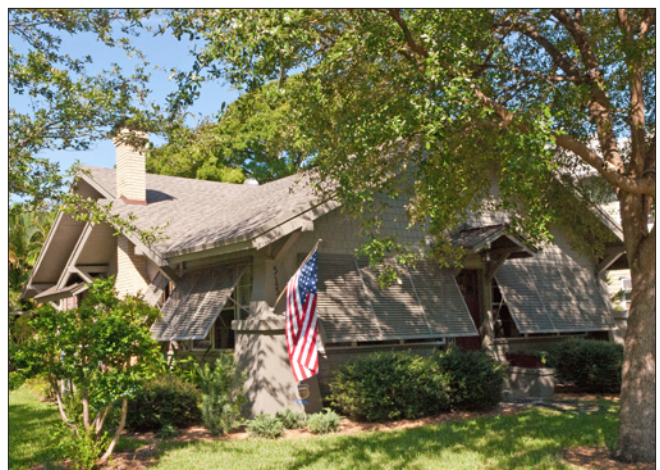
This Arts and Crafts style, wood-framed bungalow has a cross gable roof with bracketed deep overhanging eaves. Also note the tapered corner piers, typical of the style.
