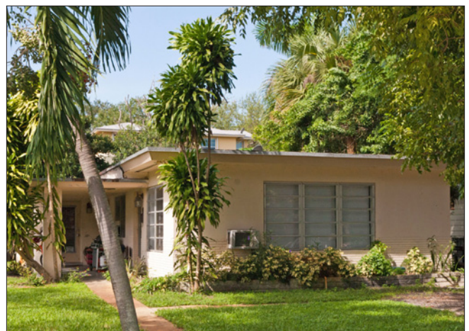
This 1-story, flat roofed, stuccoed, masonry vernacular residence has deep overhanging eaves and grouped awning windows, reminiscent of Mid-Century Modern style.
