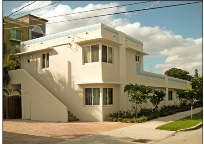
This Art Moderne building has a 2-story main block with a 1-story wing visually joined by with a decorative band. Windows wrap around corners and are covered by cantilevered sun screens.
