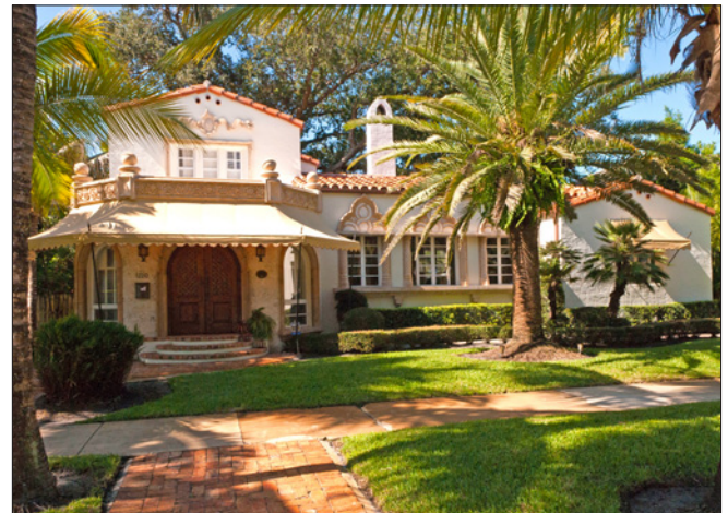
This Mediterranean Revival / Spanish Eclectic home has several stone and cast stone embellishments including the projecting entrance and window surrounds.
