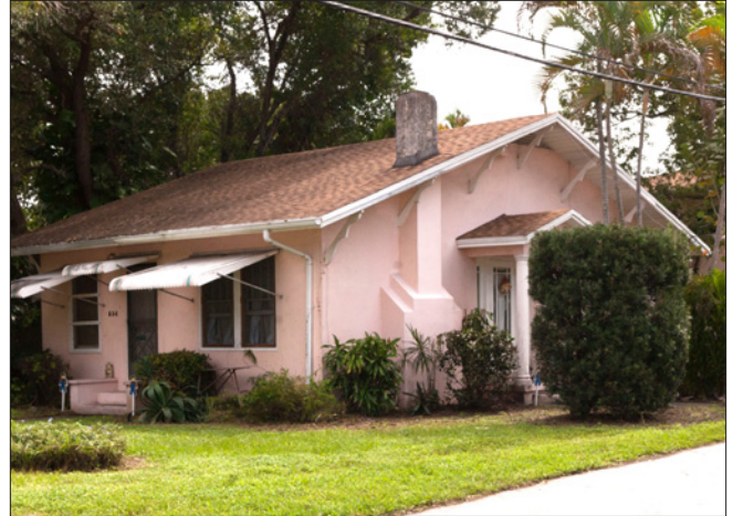
This stuccoed masonry house is 1-story in height, has a front gable roof with overhanging eaves, and has single and paired double-hung windows.
