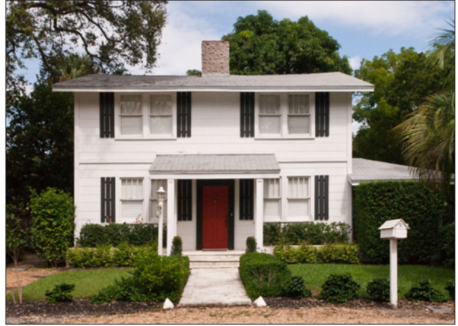
Two-story frame residences are less common than 1-story homes. This example includes a side-gable roof with deep overhanging eaves and paired 4-over-1 double-hung windows.
