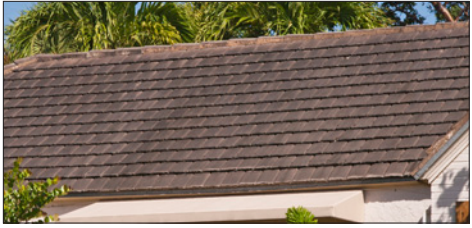
Tile roofing is available in a variety of profiles. These concrete tiles are relatively flat and are similar in appearance to slate roofing.
