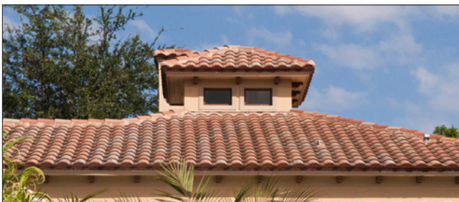
This cupola is topped by a hipped roof and includes windows at each face.
