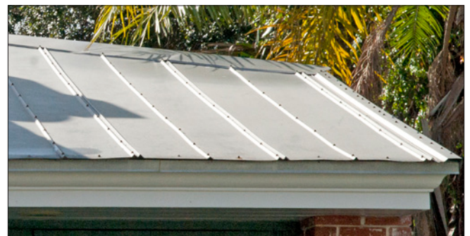
5-V crimp roofing panels were popularized in the mid to late 20th century. They can provide a weather-tight roof system.
