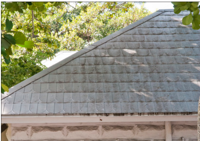
These decorative metal shingles include an embossed pattern on each shingle that adds to the roof's texture.
