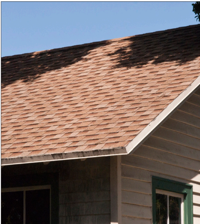
Asphalt shingles often replicate alternate materials such as wood shingles.
