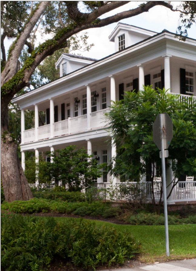
Historic porches - such as the multi-level porch on this historic house - can be an important element of a building's exterior.
