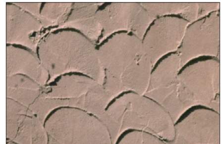
Trowel Finish Stucco - Highly stylized finish with pronounced ridges and shadows from trowel application.
