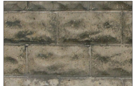
Rusticated Concrete Block - A structural building material made by mixing water, cement, sand and aggregate, placing it in forms and hardening; commonly used for foundations, walls and piers, popular in the early to mid 20th century.
