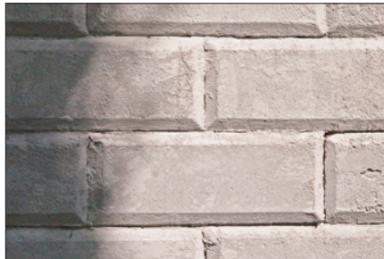
Textured Concrete Block - A structural building material made by mixing water, cement, sand and aggregate, placing it in forms and hardening; commonly used for foundations, walls and piers, popular in the early to mid 20th century.
