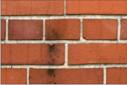
20th Century Brick - A hard, dense, fired-clay, regularly shaped building component; sometimes with a glazed surface; used primarily in walls, piers, foundations and exterior pavers.
