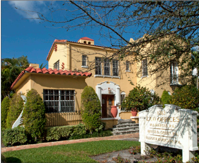
Stucco is a versatile material that is used in a variety of architectural styles, such as this Arbreu designed house, now used as offices.
