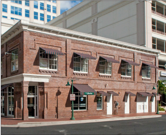
While uncommon, there are several brick buildings in Fort Lauderdale. The Shepard Building represents one of the oldest brick buildings in the City. It includes several decorative brick details including: horizontal banding between the first and second floors; pilasters and piers; corbelling below the main cornice; and projecting trim framing the top of the second floor windows with bracketed projecting sills.
