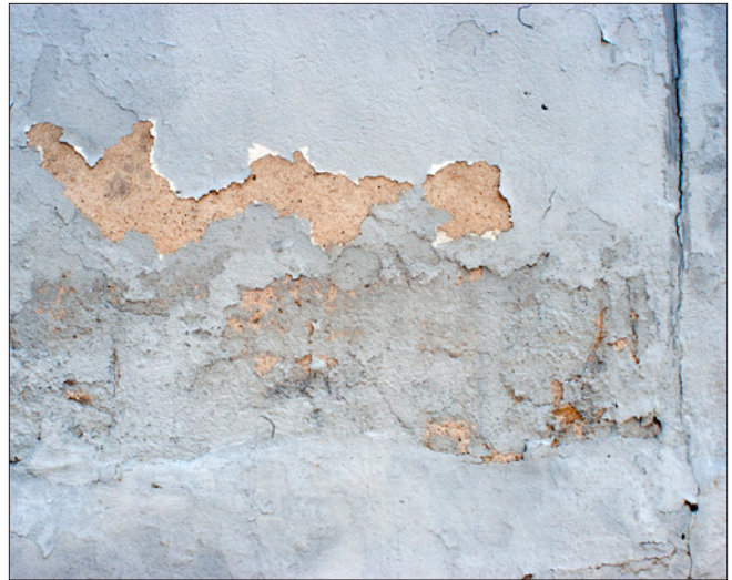
When painting stucco, it is recommended that a breathable masonry paint be used and that loose or flaking paint be removed prior to repainting.
