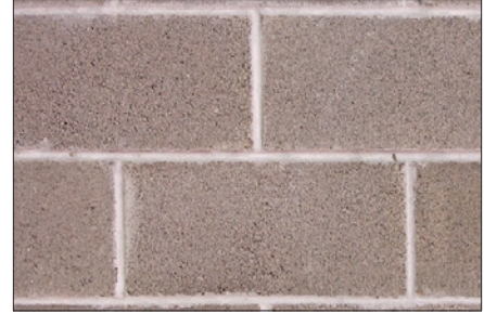
Concrete Block - A structural building material made by mixing water, cement, sand and aggregate, placing the mix in forms and hardening; commonly used for foundations, walls and piers.
