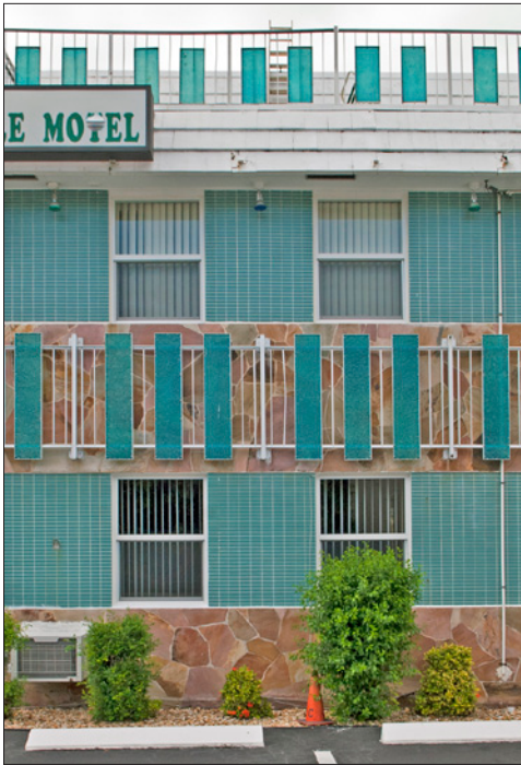
This concrete framed building has applied glazed-tile, stone veneer, and acrylic panels on a metal framework.
