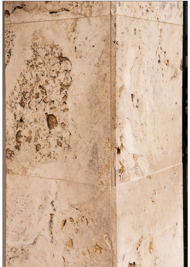
Stone veneer, such as this oolite example, consists of thin slabs of stone that are "hung" from an underlying structural system.
