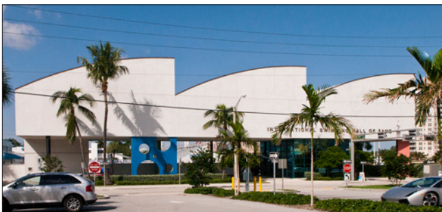
Concrete is a versatile material that can be used to create complex forms and shapes.
