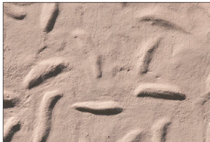
Textured Stucco - A distinctive, raised stucco finish used in buildings designed by Abreu.
