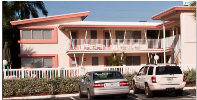
This Mid-Century Modern motel includes metal railings, diagonal “beanpoles” and a metal post to the right supporting the corner of the roof overhang.
