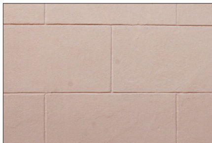
Scored Stucco - Smooth finish with scoring to simulate stone joints.
