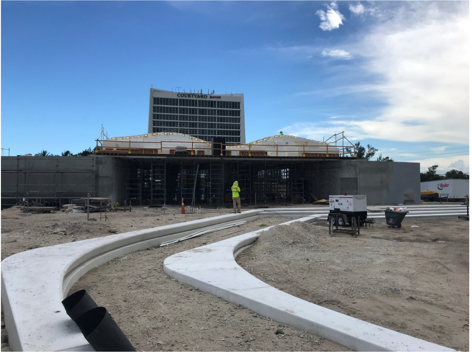
OCEANSIDE PARK PROGRESS PHOTO TAKEN ON 7-30-2019 (VISITOR CENTER/BATHROOM BUILDING)
