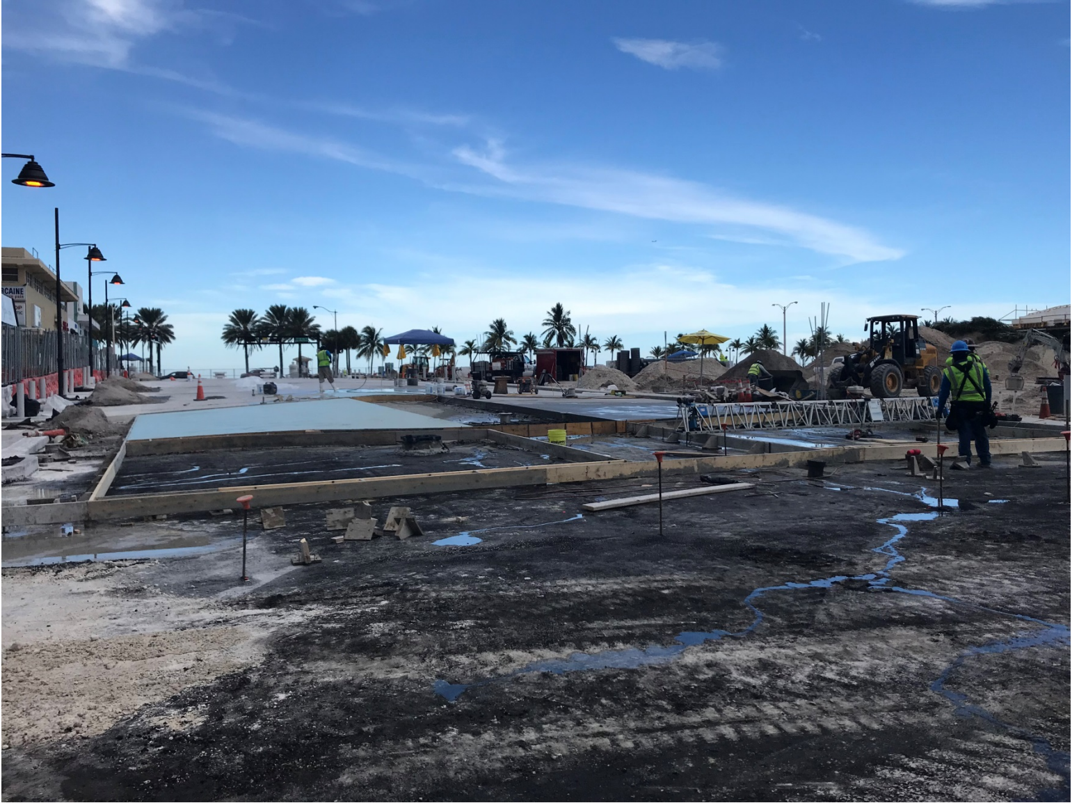
FESTIVAL STREET PROGRESS PHOTO TAKEN ON 7-30-2019 (LAS OLAS BLVD FACING EAST)
