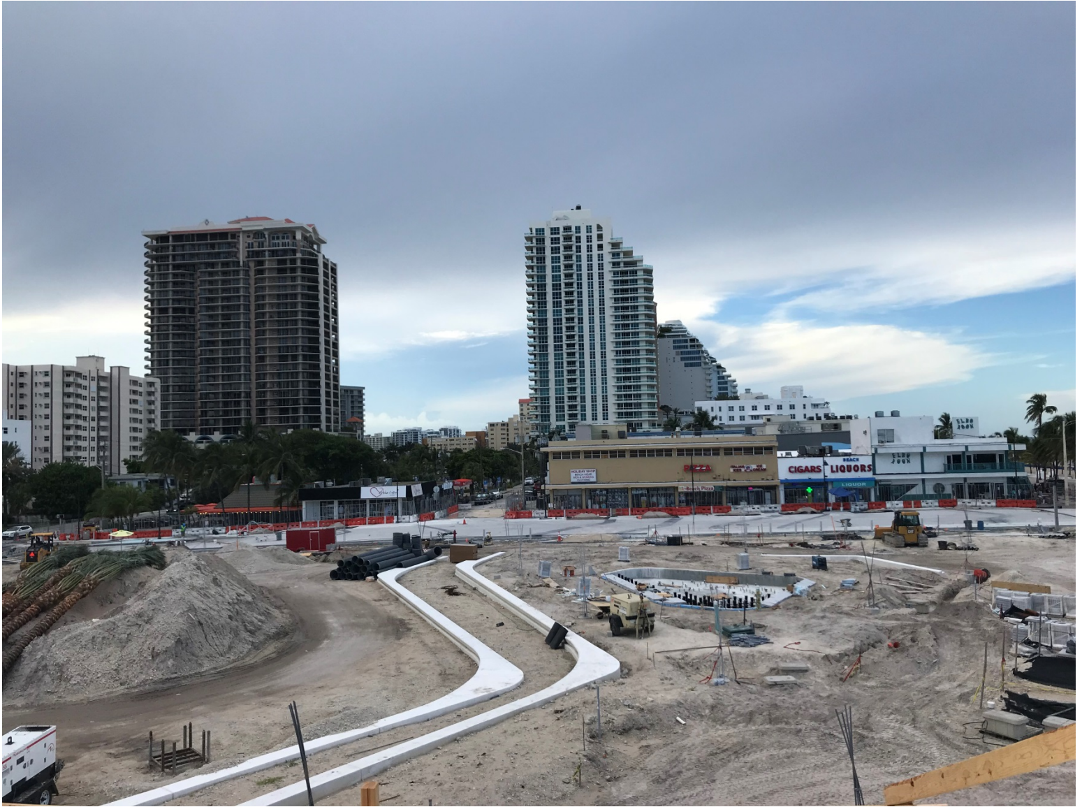
OCEANSIDE PARK PROGRESS PHOTO TAKEN ON 7-30-2019 (FACING NORTH)
