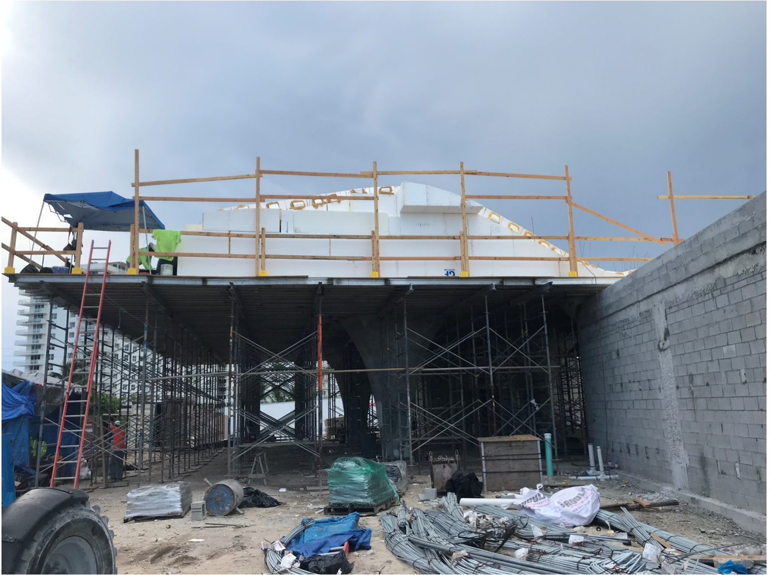
OCEANSIDE PARK PROGRESS PHOTO TAKEN ON 7-30-2019 (SHADE CANOPY)
