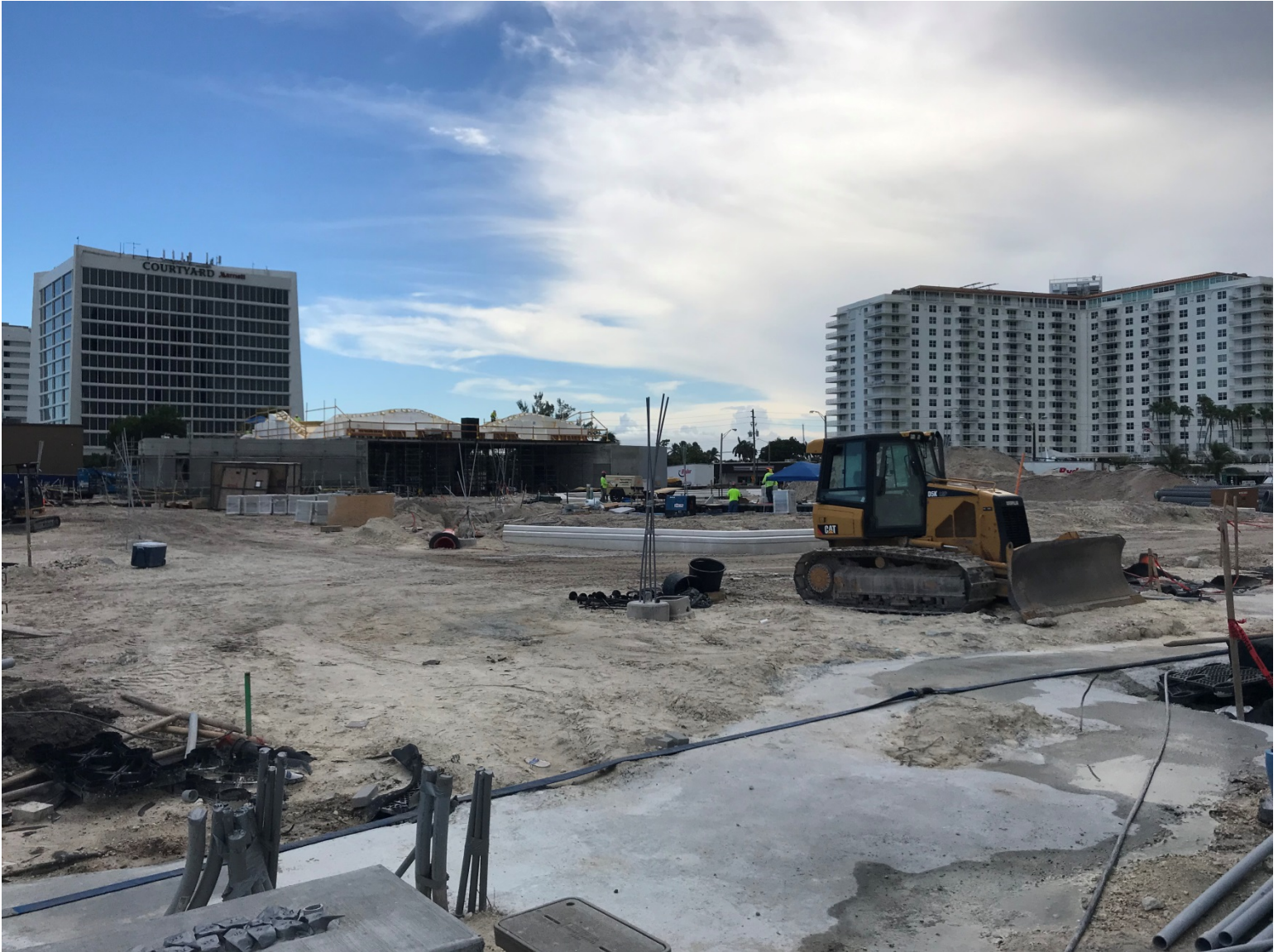
OCEANSIDE PARK PROGRESS PHOTO TAKEN ON 7-30-2019 (FACING SOUTH)
