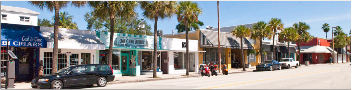
Rows of storefronts generally share common features including large display windows along the ground floor that allow pedestrians to see within, and a band of signs and awnings at a fairly consistent height along a streetscape.
