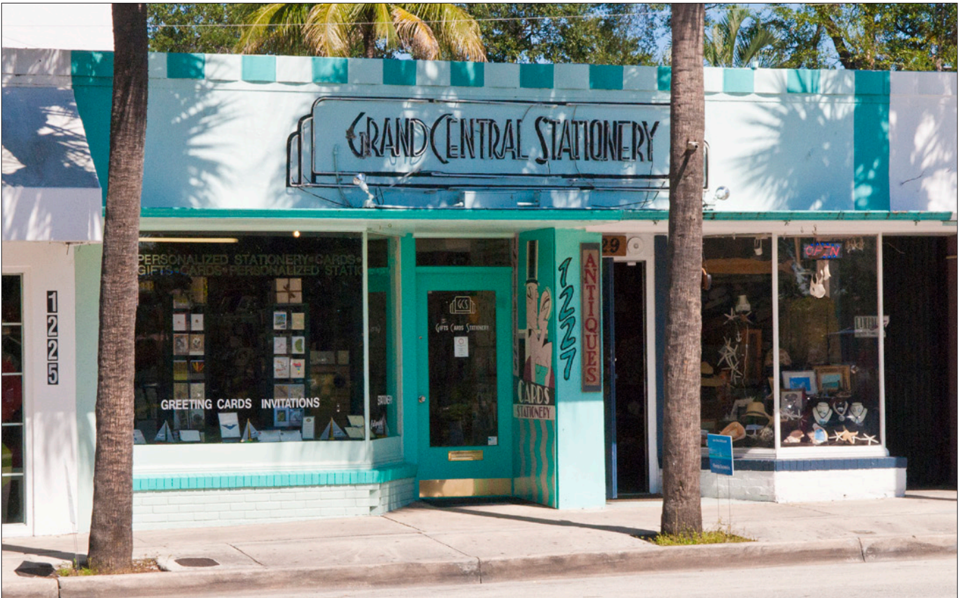
This storefront includes large display windows, a entrance alcove with a wood, single-light door topped by a transom window, a customized neon sign and a unique paint scheme that complements its architectural style.
