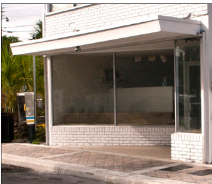
The storefront cornice at this Mid-Century Modern building projects far enough to act as an awning, providing protection for customers and display merchandise. The entrance alcove increases the visibility of storefront displays.
