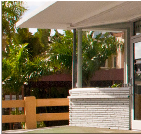
Although most structural supports are incorporated into the window frame system, in this example a pole is located inside the corner of the glass.
