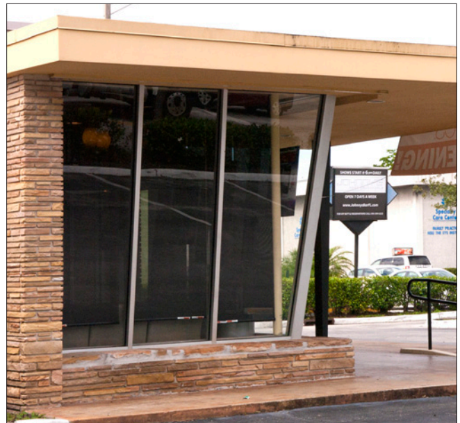
Canted or angled display windows are often found at Mid-Century Modern buildings and should be preserved.
