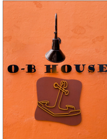
A single gooseneck light illuminates this pin-mounted wall sign. The conduit for the light and mounting connections for the signage have been concealed.
