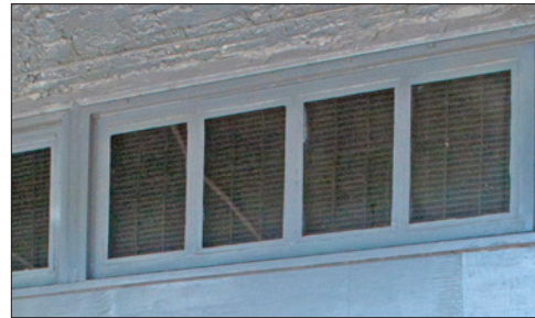
These multi-light wood transom windows are located above the operable, wood storefront doors with similar divided lights.
