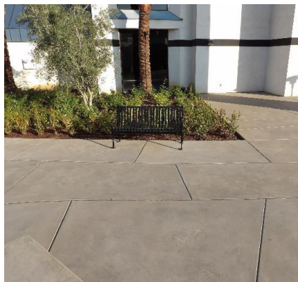
Sidewalk Tinted & Scored Concrete in three tones
