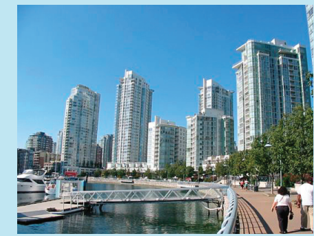
Buildings are slender, and their narrowest dimensions are oriented parallel to the water's edge to allow air, views and greater space between them along the Vancouver, Canada waterfront
