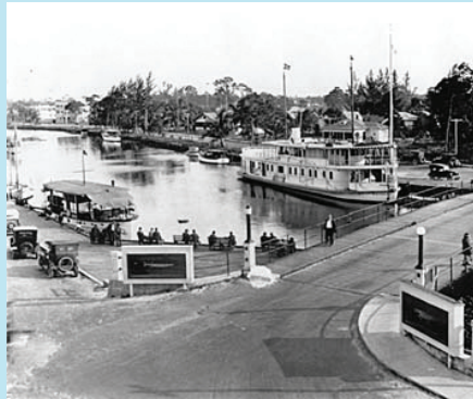
A historical photo of Andrews Avenue Bridge, showing that the bridge was once at grade level allowing convenient pedestrian crossing
