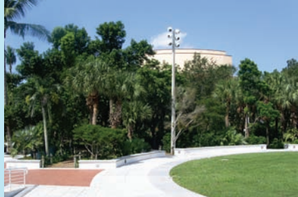
Existing conditions: PAC is detached from the park, separated by berms and landscaping: no 'eyes on the park' to encourage feeling of activity and safety
