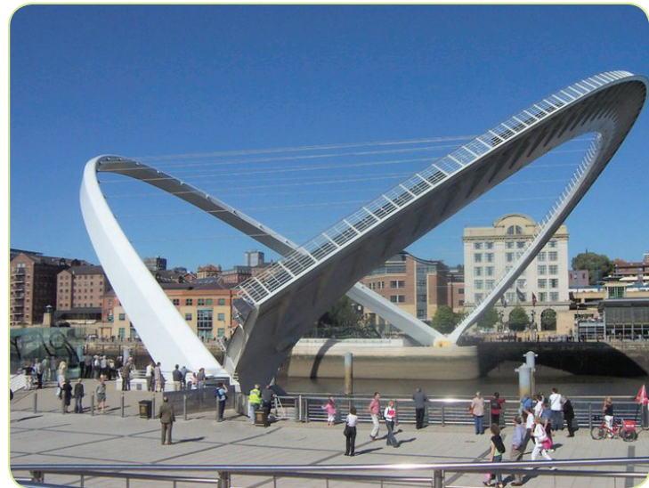
Gateshead Millennium Footbridge, London
