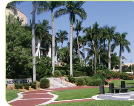
Existing Conditions: Densely landscaped hillside separates the Broward Center of Performing Arts from Esplanade Park, blocking views from the PAC towards the river, and adding to the feeling of isolation and lack of safety in the park at night
