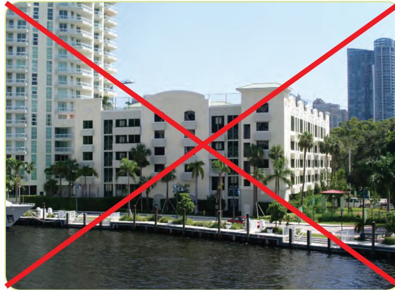
Existing parking garage on the river
