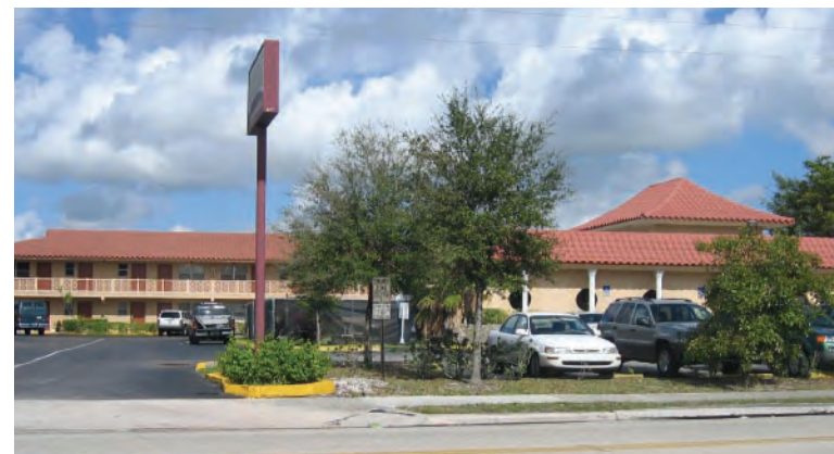
Office along Davie Boulevard near I-95.
