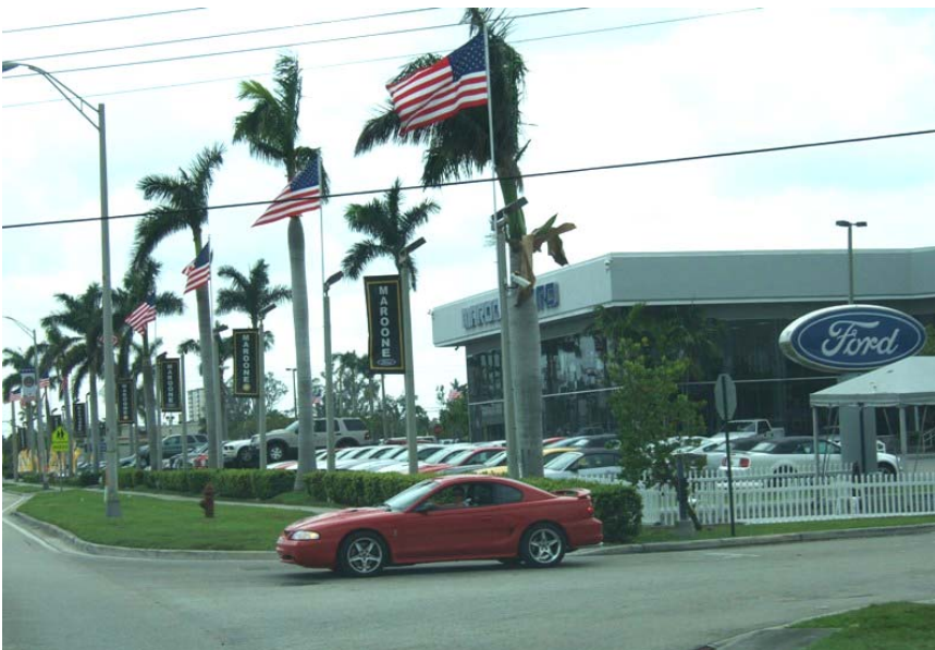
Figure 3.28: Traditional auto dealerships account for a majority of the land area within the Gateway district, with large sites being of sufficient size to accommodate future mixed-use redevelopments.
