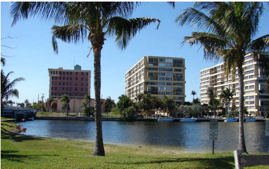
Figure 3.27: A view from George English Park across the Middle River shows the opportunity for large-scale mixed-use redevelopment with waterfront destination activity.
