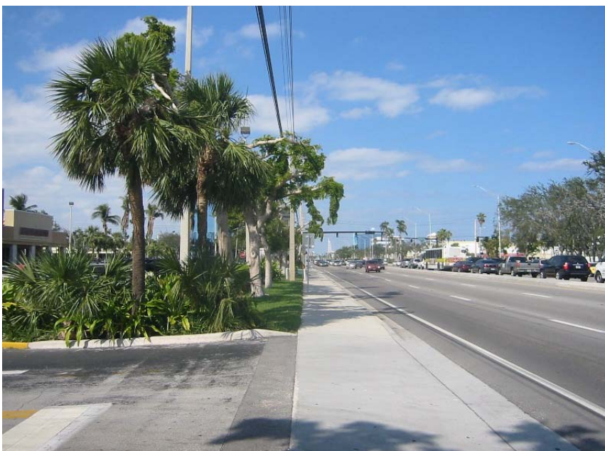
Figure 2.7: Typical sidewalk adjacent to curb with no buffer between pedestrian and fast moving vehicles
