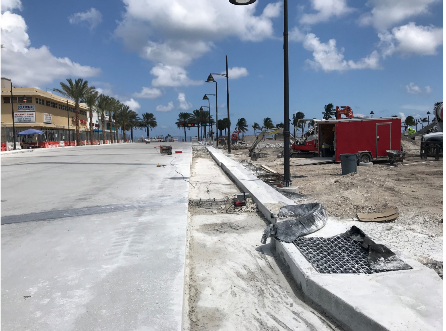
FESTIVAL STREET PROGRESS PHOTO TAKEN ON 9-11-2019 (LAS OLAS BLVD FACING EAST)
