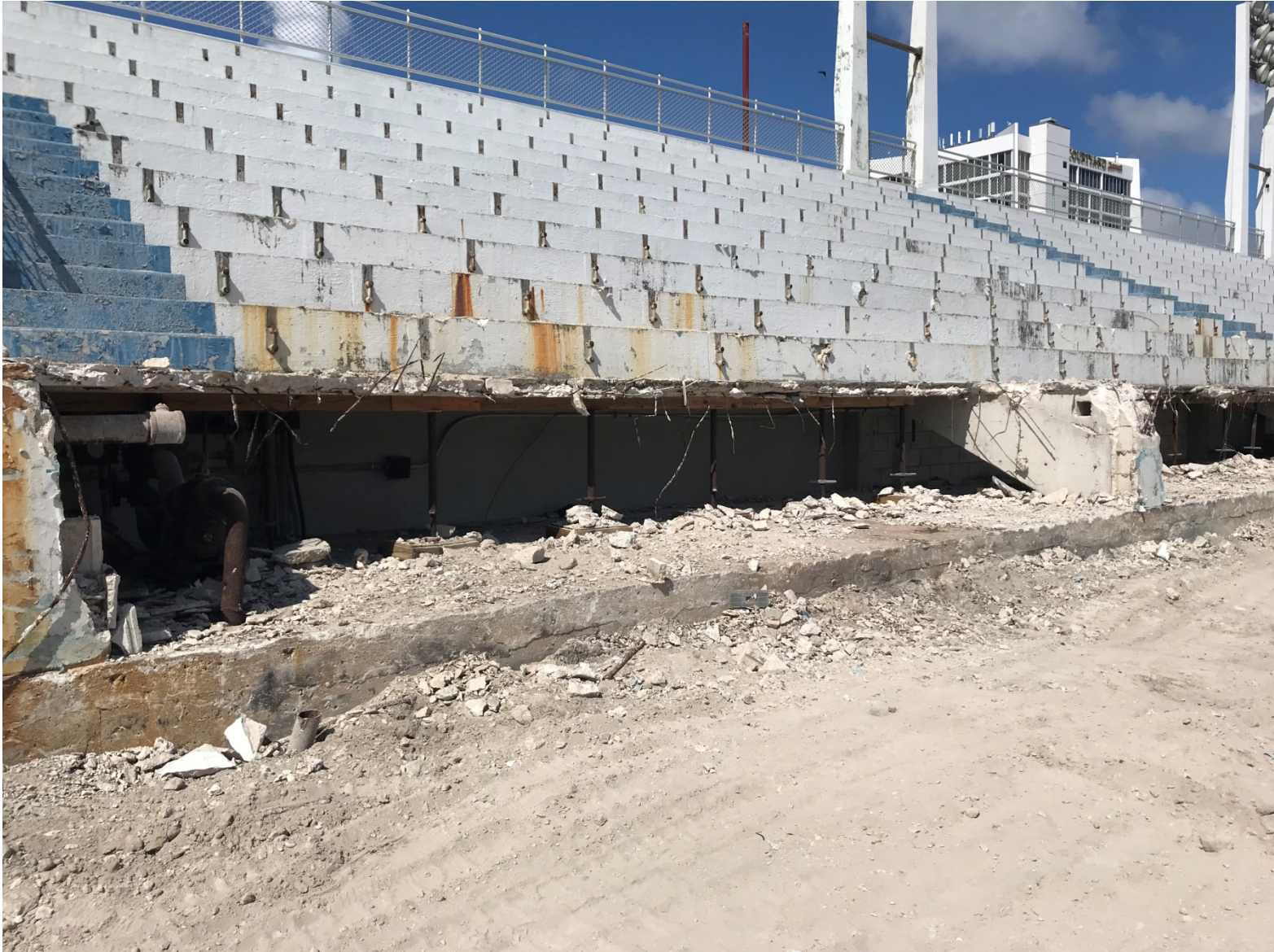
AQUATIC CENTER PHOTO TAKEN ON 9-10-2019 (FACING NORTH – GRANDSTAND DEMOLITION)
