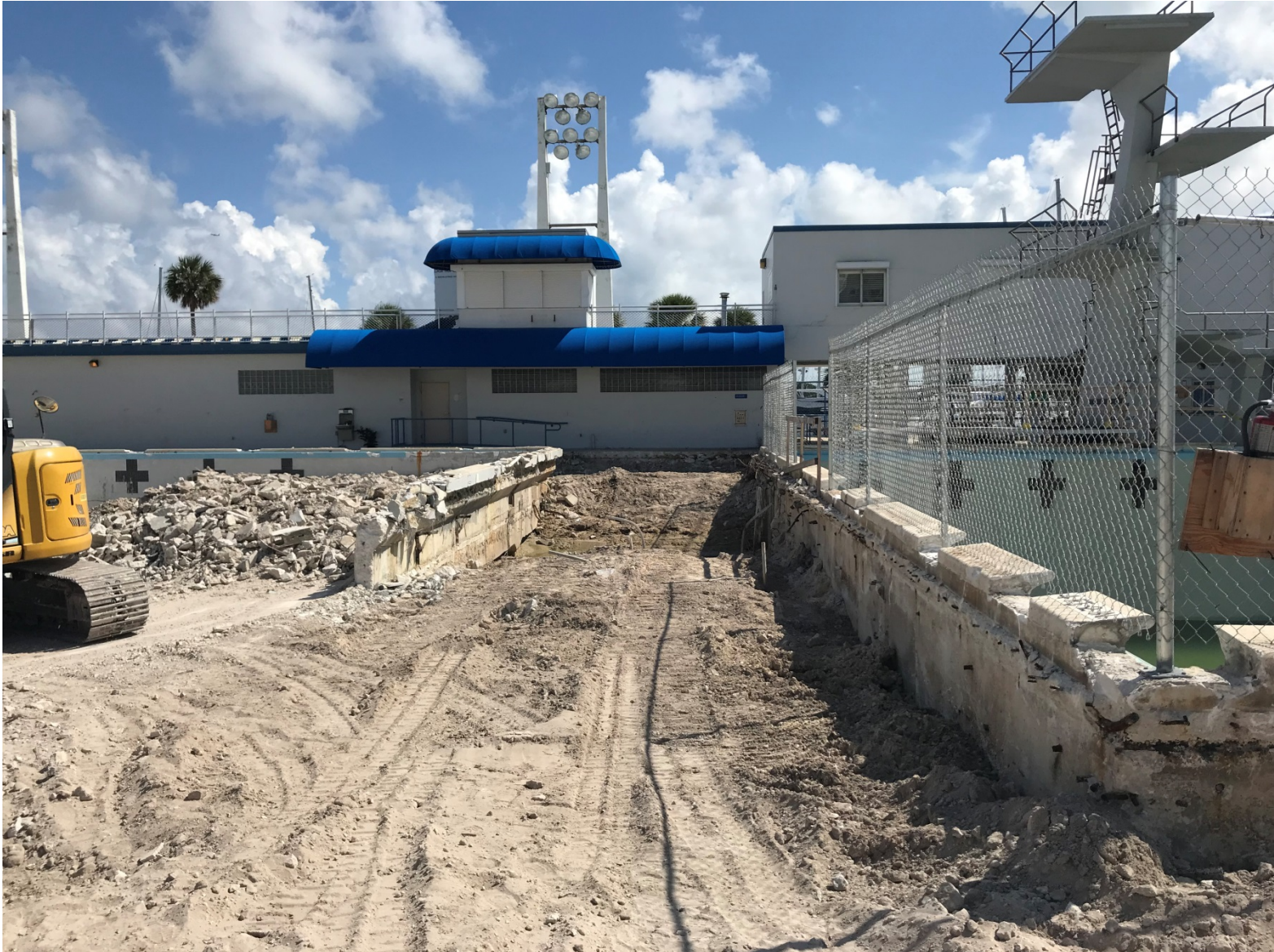
AQUATIC CENTER PHOTO TAKEN ON 9-10-2019 (FACING SOUTH – POOL DECK DEMOLITION)
