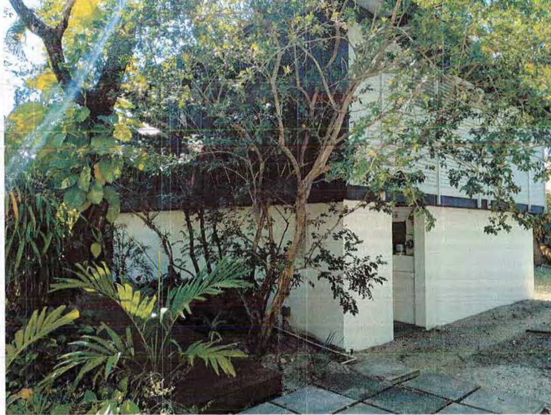
SIDE OF HOUSE, FACING SOUTH
