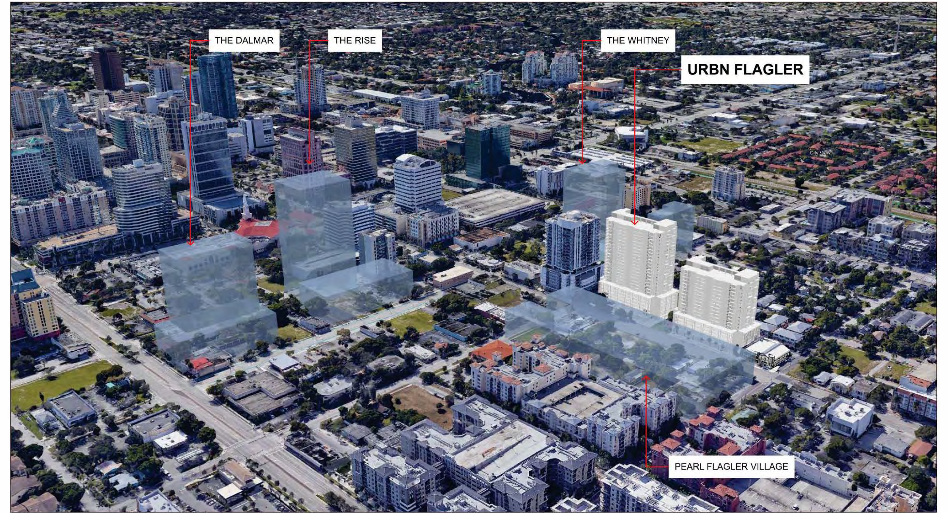
CONTEXT VIEW SOUTHWEST
