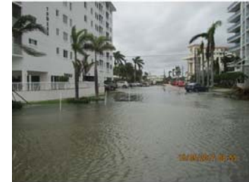
Bayshore Drive Before Improvements
