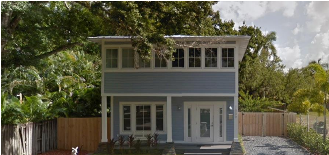
Front Façade of Main House on Site
