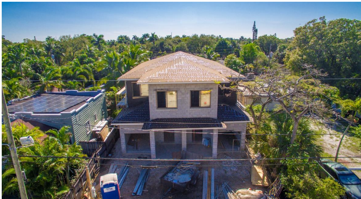
Current Condition of New Construction Project
