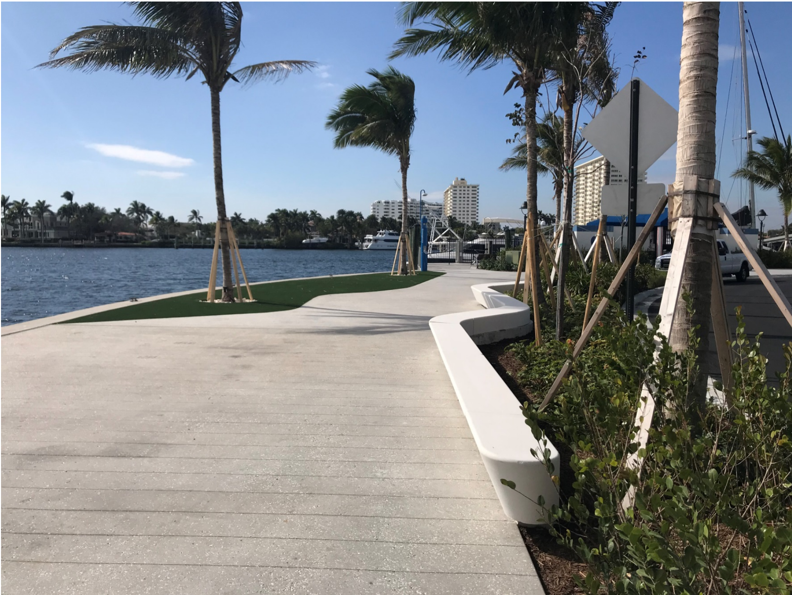
LAS OLAS PROJECT PROGRESS PHOTO 1-22-2020 (SEATWALL AND ARTIFICIAL TURF INSTALLATION)
