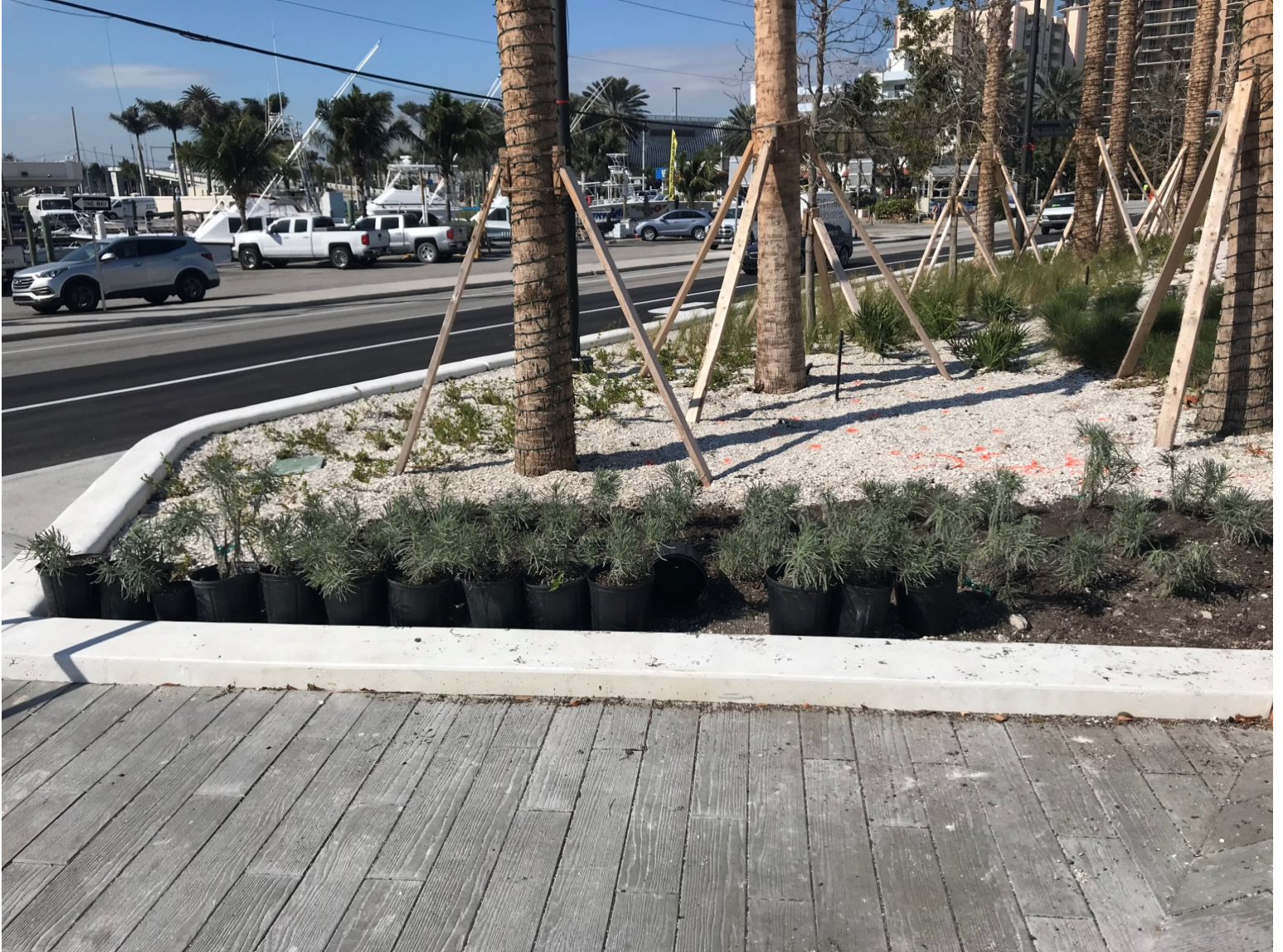
LAS OLAS PROJECT PROGRESS PHOTO 1-22-2020 (INSTALLATION OF DUNE SHRUB PLANT MATERIAL)
