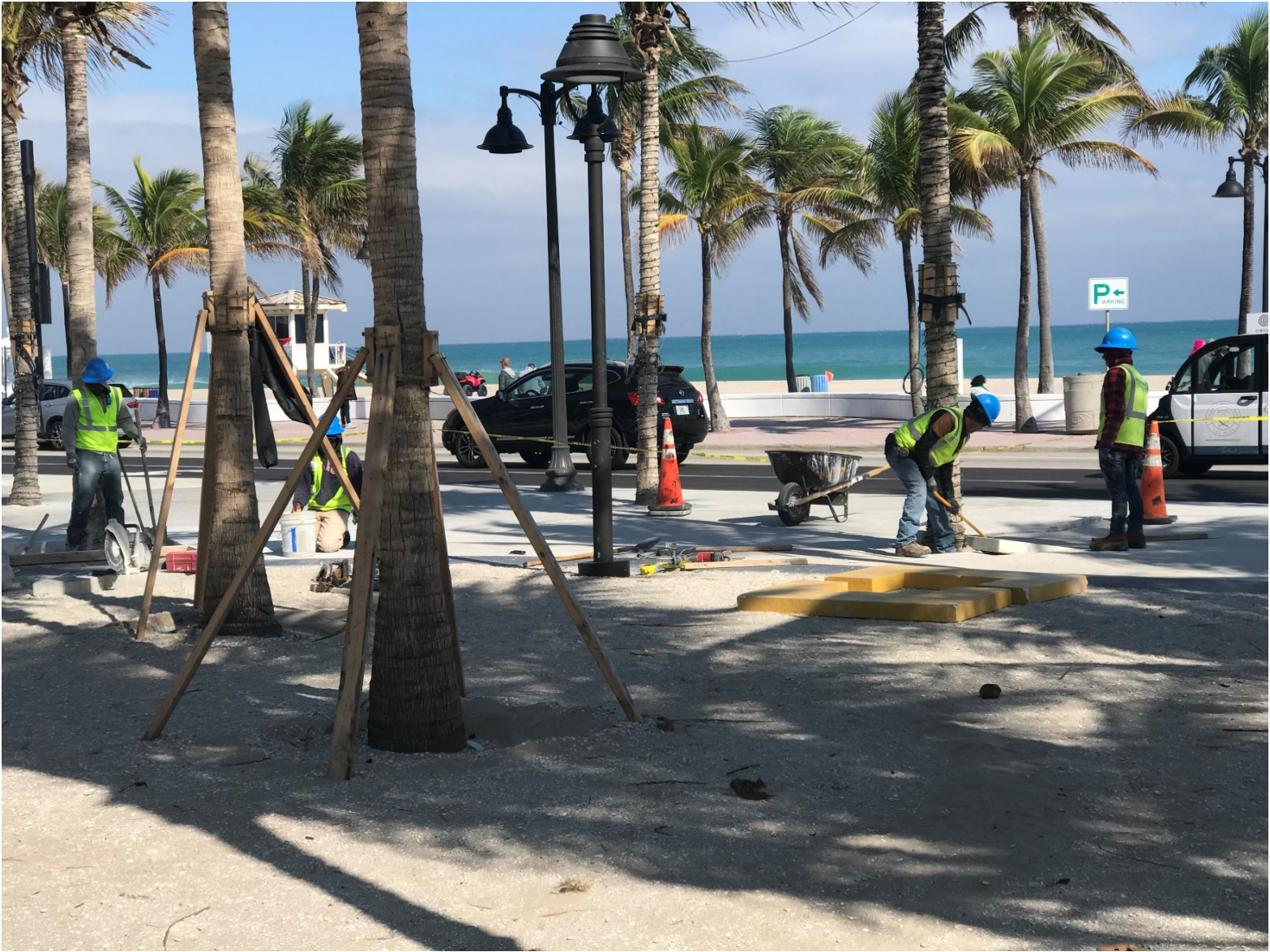
LAS OLAS PROJECT PROGRESS PHOTO 1-22-2020 (SETTING AND ADJUSTING TREE GRATE FRAMES)
