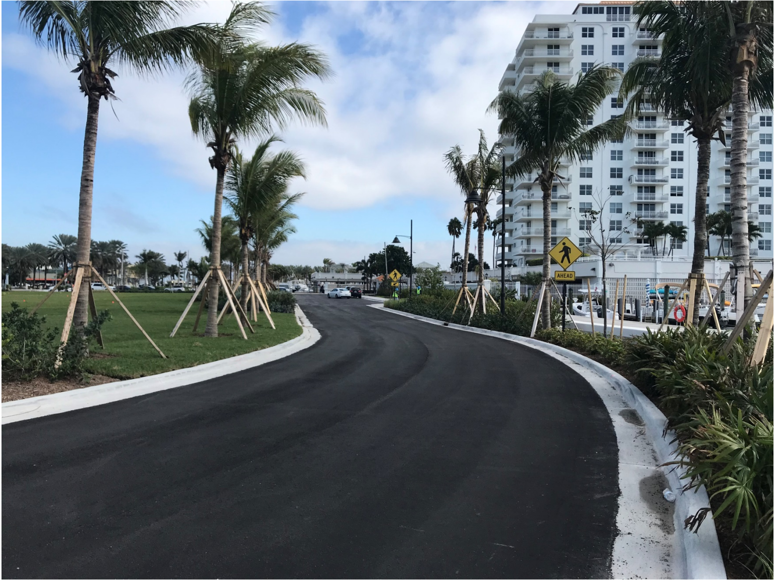
LAS OLAS PROJECT PROGRESS PHOTO 1-22-2020 (ASPHALT INSTALLATION)
