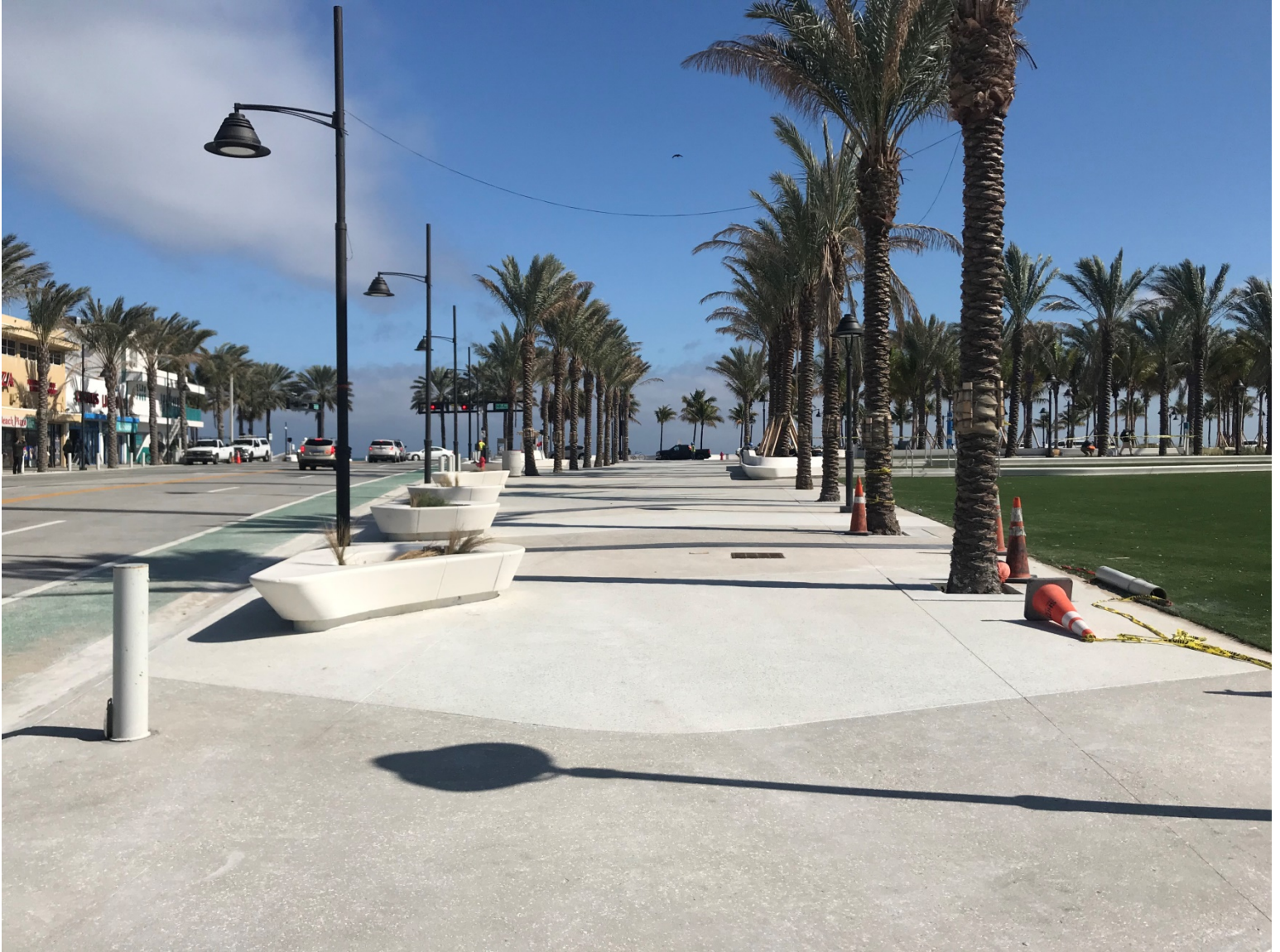
LAS OLAS PROJECT PROGRESS PHOTO 1-22-2020 (SIDEWALK PUNCH WORK COMPLETION)
