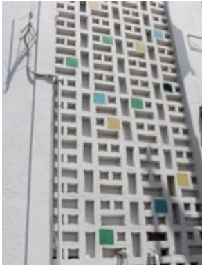
Concrete screen block
