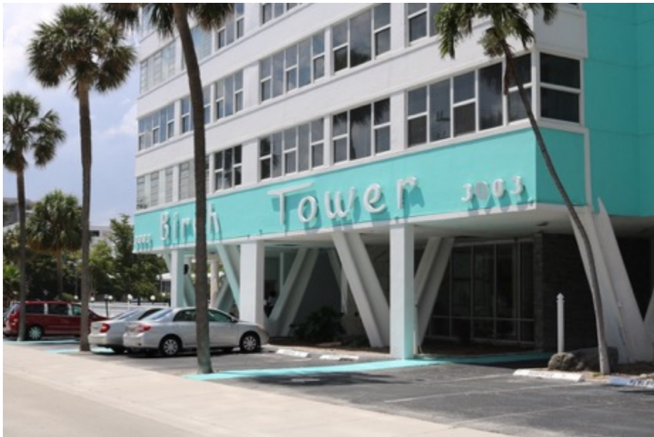
Image 16: Birch Tower South Façade, Looking North West Photo: Morris Hylton III, April 19, 2019
