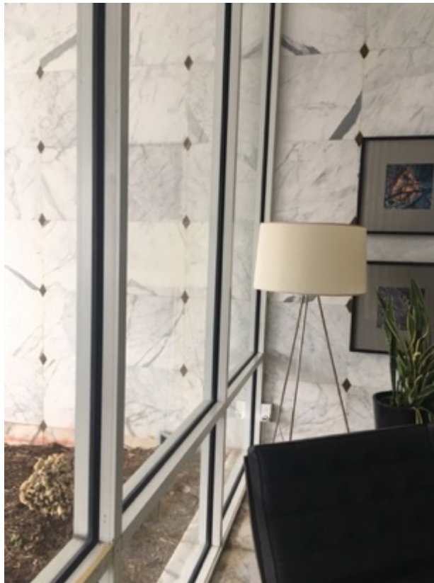
Image 22: Birch Tower, Lobby, West and South Walls, Looking South-West Photo: Morris Hylton III, April 19, 2019
