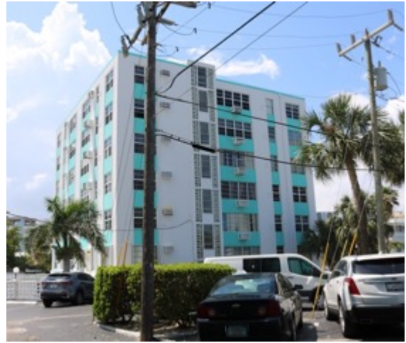
Image 37: Birch Square, Parking Lots, Looking North-West Photo: Morris Hylton III, April 19, 2019
