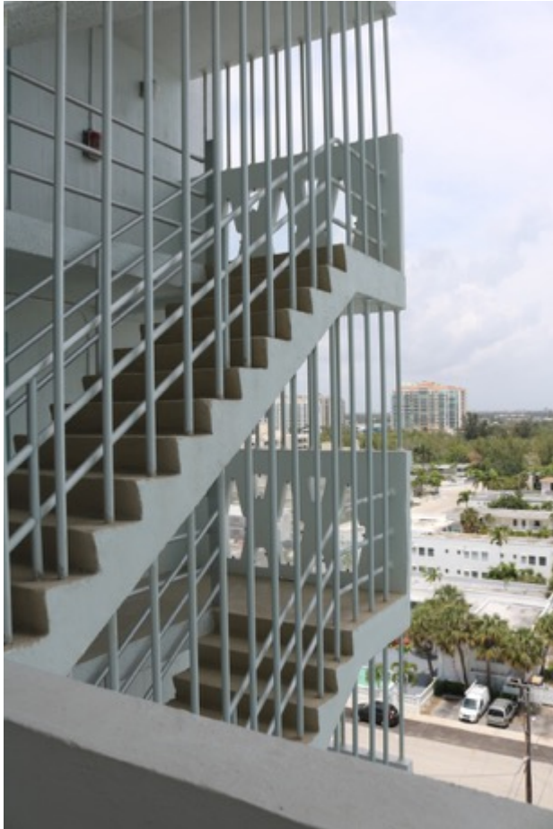
Image 30: Birch Tower, North Stairs, Looking North-East Photo: Morris Hylton III, April 19, 2019
