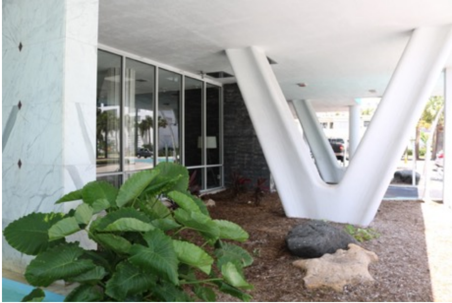
Image 17: Birch Tower, South Façade, Looking East Photo: Morris Hylton III, April 19, 2019
