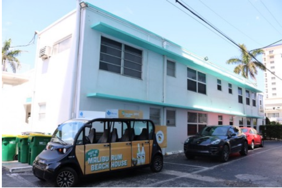
Image 3: Birch Terrace, South Façade, Looking North-East Photo: Morris Hylton III, April 19, 2019
