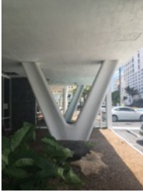
Concrete pilotis
