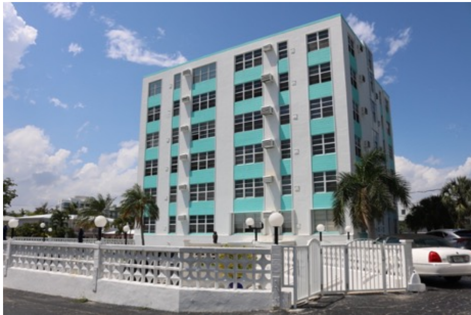
Image 14: Birch House, South Façade, Looking North-East Photo: Morris Hylton III, April 19, 2019
