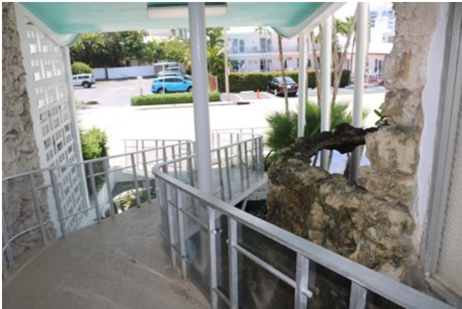
Image 10: Birch House, Main Entrance Looking West Photo: Morris Hylton III, April 19, 2019
