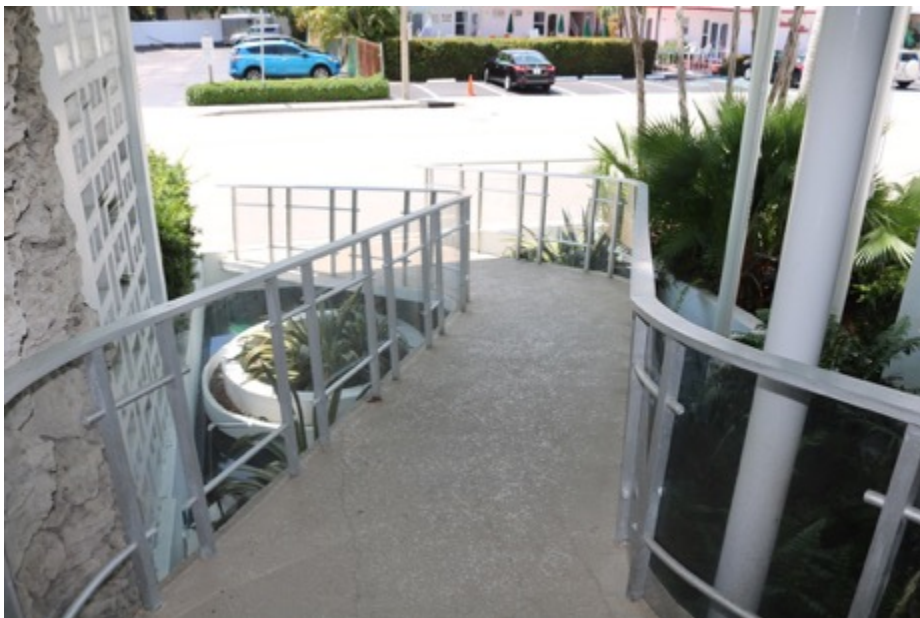
Image 8: Birch House, Main Entrance Looking North-West Photo: Morris Hylton III, April 19, 2019
