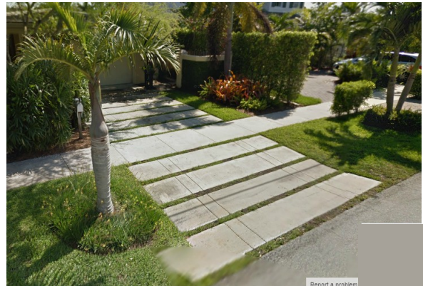
Segmented Concrete Driveway 1600 block NE 5th Street
