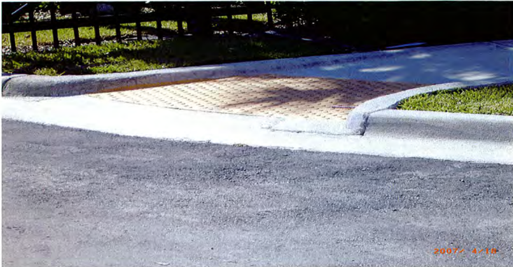
Picture 1: Fort Lauderdale Building Services, 700 N.W 19 th Avenue Fort Lauderdale
