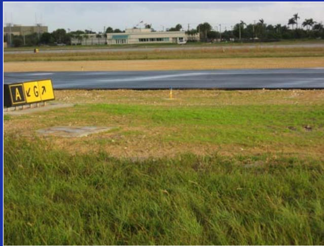
Relocation of Taxiway Golf Phase I
