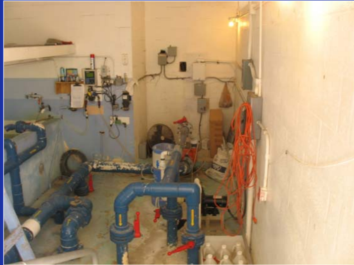
Pool Equipment Replacements
