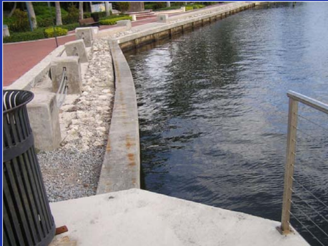
Marine Facility, Seawall and Mooring Buoy Renovations
