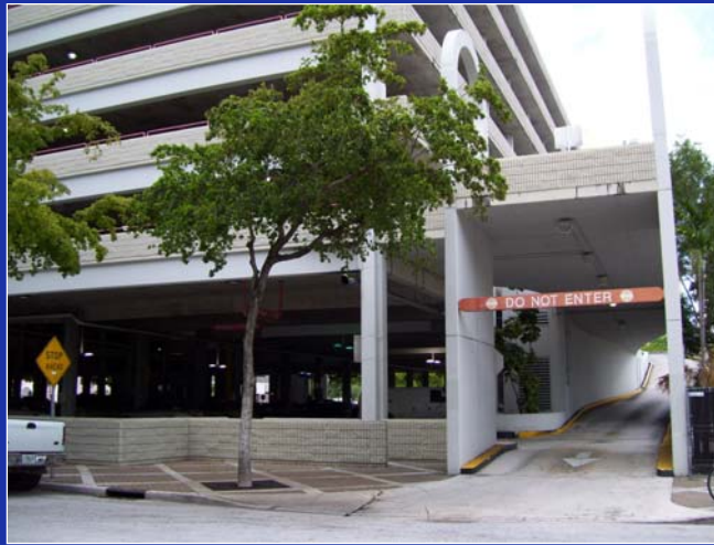
City Park Garage Phase 3- Facade/Signage
