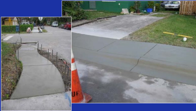
Concrete Sidewalk- Sunrise Boulevard to NW 12 Street
