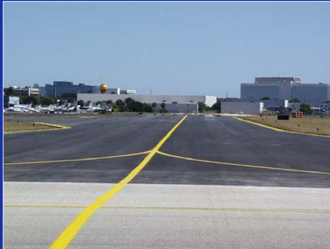
Taxiway C & D Pavement Rehabilitation
