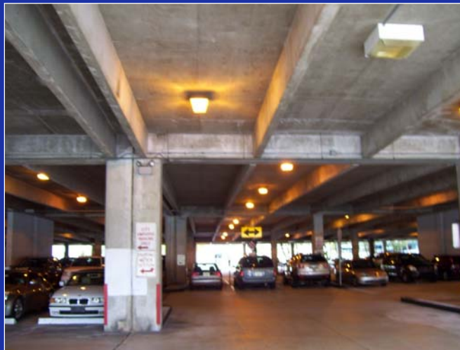
City Hall Garage Lighting Rehab
