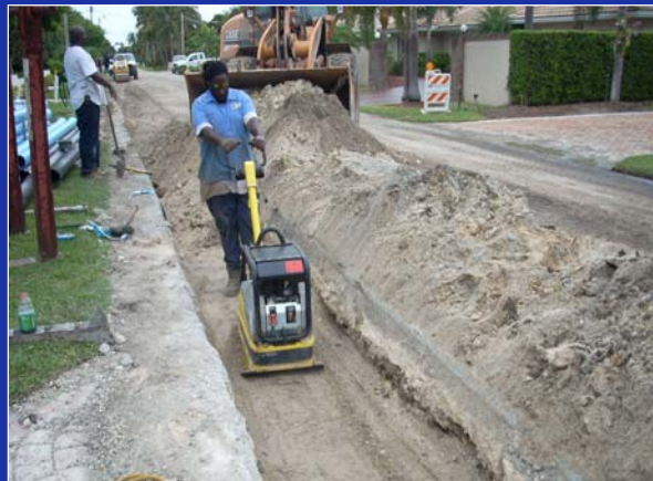
Small Water Main Replacement
