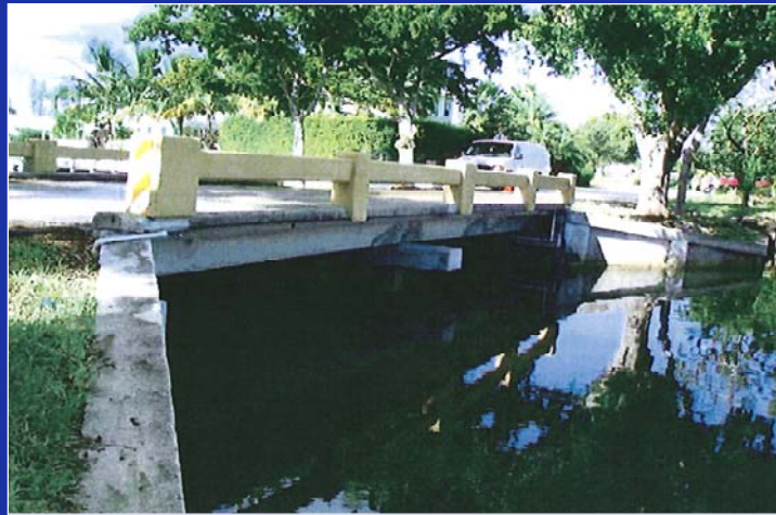
Bridge Repairs at Several Locations
