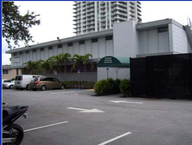
Parking Administration Building Structural Repairs
