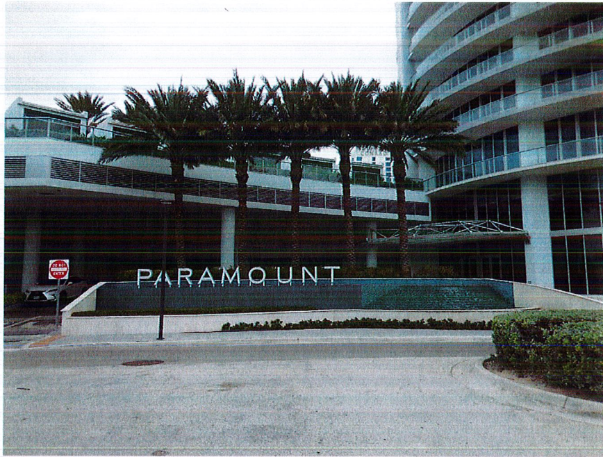
View south across Vistamar Street (towards east end)
