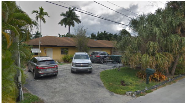
Building not visible from street, photo courtesy of Google Streetview
