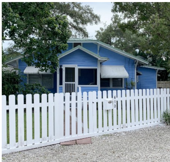
Figure 6B-4: The house at 610 SW 5th Place is an example of the Craftsman style. Photo by Trisha Logan.
