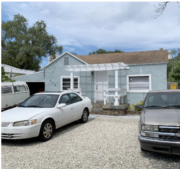
Figure 6B-6: The house at 528 SW 5th Avenue is an example of the Minimal Traditional style. Photo by Vagabond Consulting Group.
