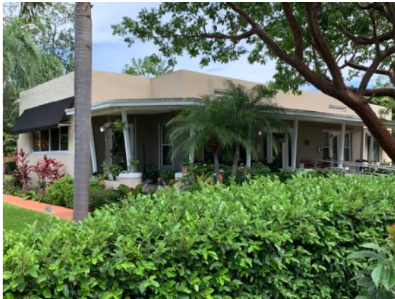
Figure 6B-8: The house at 500 SW 6th Avenue is an example of the Art Moderne style. Photo by Trisha Logan.
