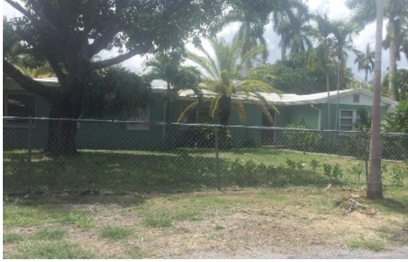
Figure 6B-11: The house at 905 Coconut Drive is an example of the Ranch style. Photo by Vagabond Consulting Group.
