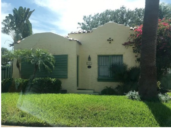
Figure 6C-7: The house at 317 NE 16th Avenue is an example of the Mission style. Photo by Vagabond Consulting Group.
