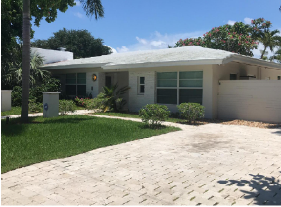
Figure 6C-11: The house at 1616 NE 8th Street designed by Lester Avery is an example of the Ranch style. Photo by Vagabond Consulting Group.
