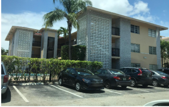
Figure 6C-13: The apartment at 1180 NE 1st Street designed by Frank Rowland is an example of the Miami Modern, or MiMo, style. Photo by Vagabond Consulting Group.
