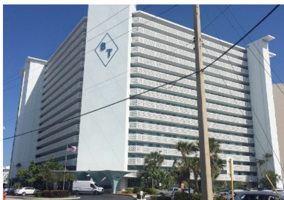
Figure 6E-5: Breakwater Towers located at 1900 S Ocean Drive is an example of the Miami Modern (MiMo). Photo by Vagabond Consulting Group.
