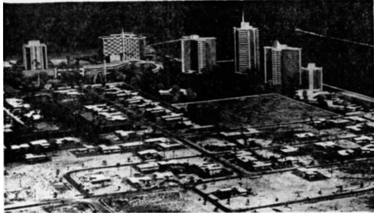
HERE'S WHAT $16,000,000 BREAKWATER BEACH DEVELOPMENT WILL LOOK LIKE WHEN COMPLETED ... Harbor Beach residential area spreads through foreground, and Port Everglades is at right center
