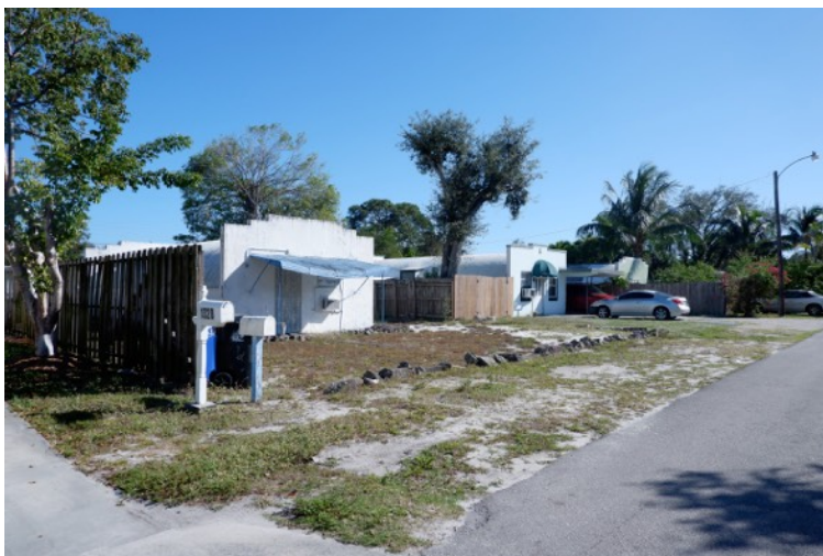
Figure 6F-2: The Quonset Huts on SW 24th Avenue were all erected in 1945. View facing south along SW 24th Avenue. Photo by Bill Morache.
