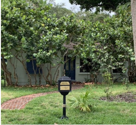
Figure 6G-8: The house at 1500 SW 13th Court, constructed in 1948, is an example of the Minimal Traditional style. Photo by Vagabond Consulting Group.
