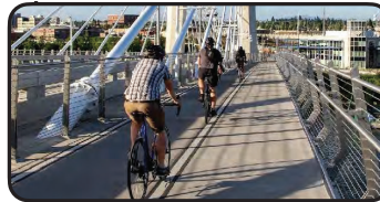
Bridge Multi-Use Paths
